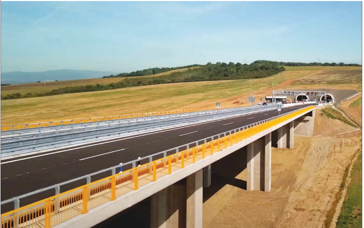
Obr. 6 Pohľad na hotový most SO 201-00, v pozadí južný portál tunela Bikoš Fig. 6 View of the completed bridge SO 201-00, with the southern portal of the Bikoš tunnel in the background
