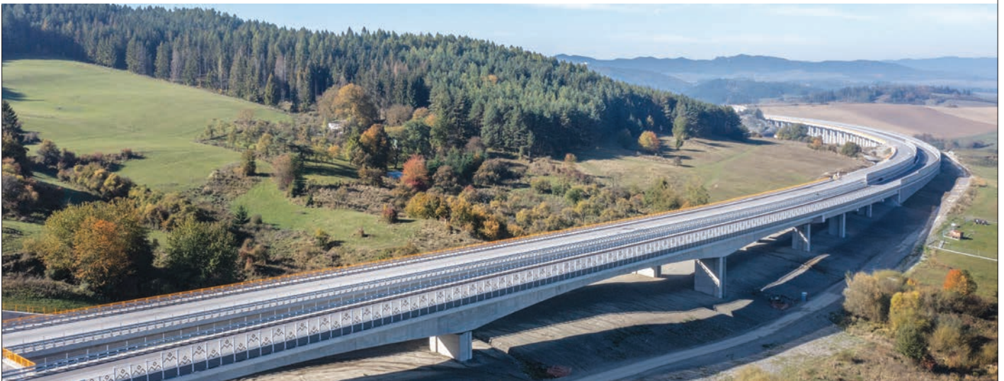
Obr. 1 Most 204 Fig. 1 Bridge 204
