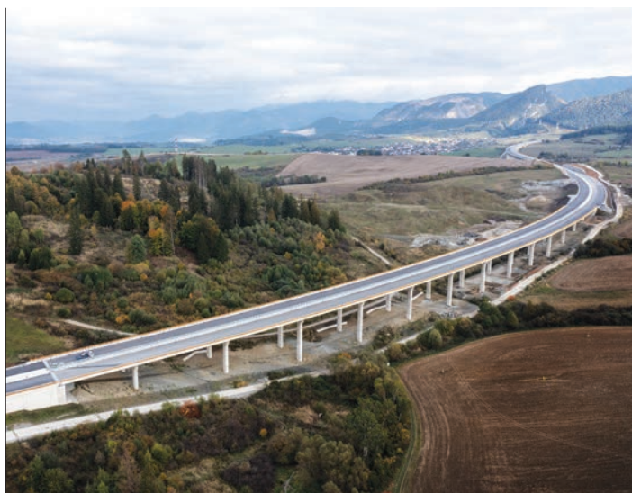
Obr. 1 Most 202 Fig. 1 Bridge 202
