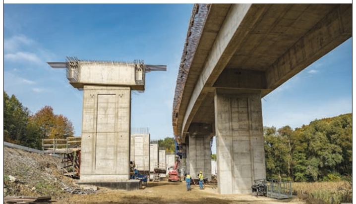
Obr. 4 Pohľad na pier s priečnikom Fig. 4 View of a pier with a crossbeam
