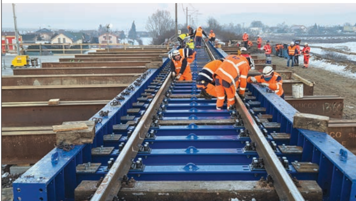
Obr. 6 Montáž stuženia koľajovej trate Fig. 6 Installation of railway track stiffness reinforcement
