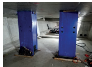
FIG. 6 Vista dos pulling sticks. View of pulling sticks.
