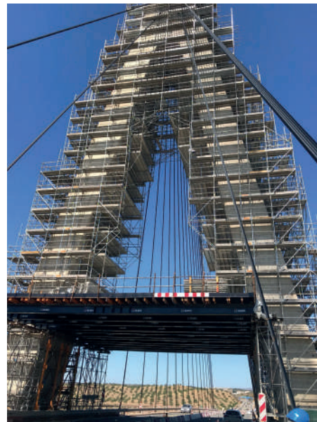
FIG. 2 Vista torre durante reabilitação. General view of the tower during rehabilitation.
