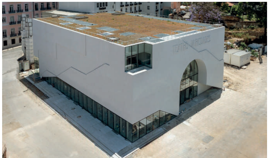
FIG. 6 Vista aérea na fase final da obra. Aerial view near completion of the works.
