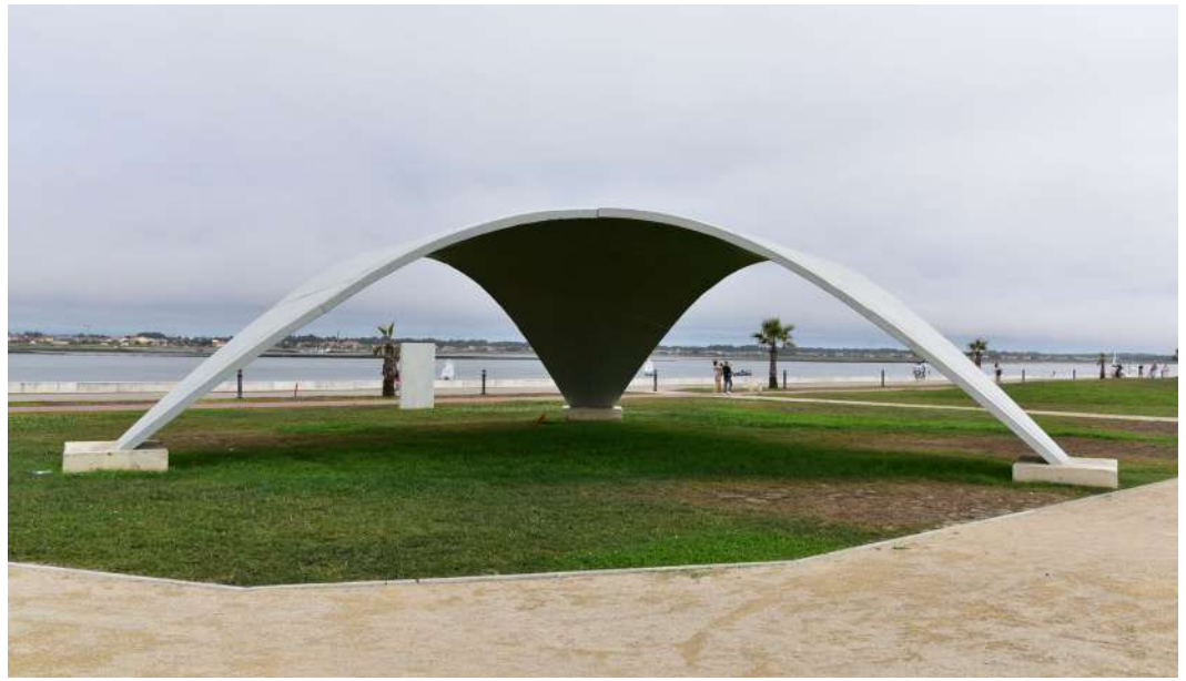
Protótipo instalado na Costa Nova, Ílhavo, Portugal – Forma final. Shell prototype in Costa Nova, Ílhavo, Portugal – Final form.
