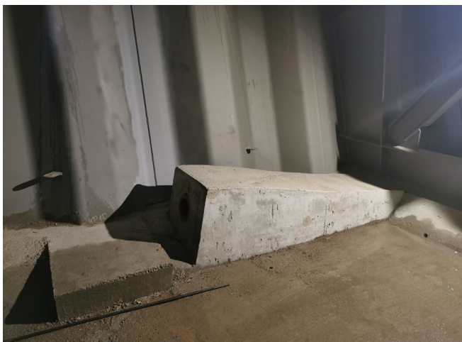
Fig 15: RC anchorage block at the bottom slab
