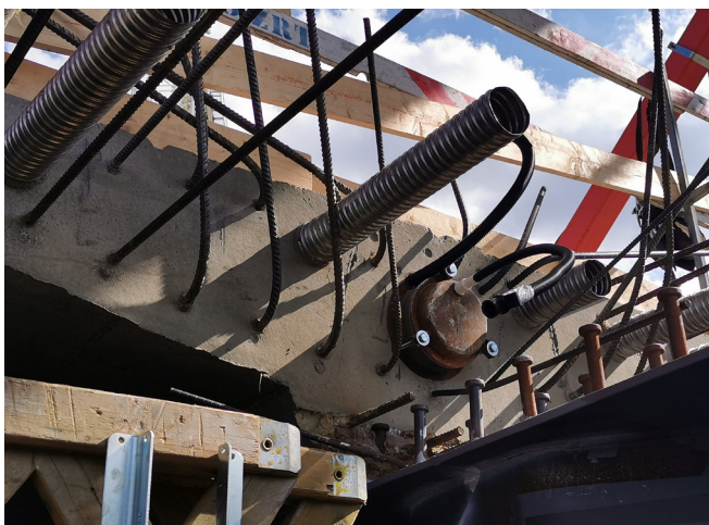
Fig 13: Post-tensioned cable anchorage in the deck slab
