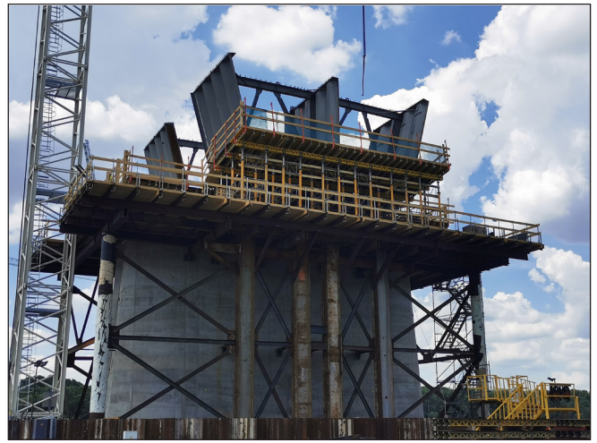
Fig 10: First segment and its auxiliary structure on the river pier
