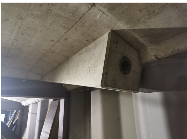
Fig 14: RC anchorage block at the deck slab
