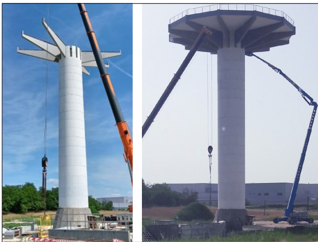
Fig. 5: The 1500 m 3 water tower in Komárom during construction
