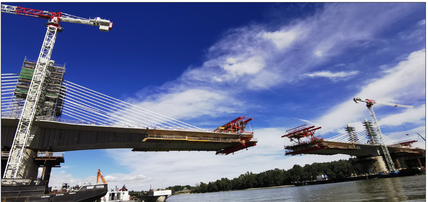
Fig 9: Free cantilevering in the main span
