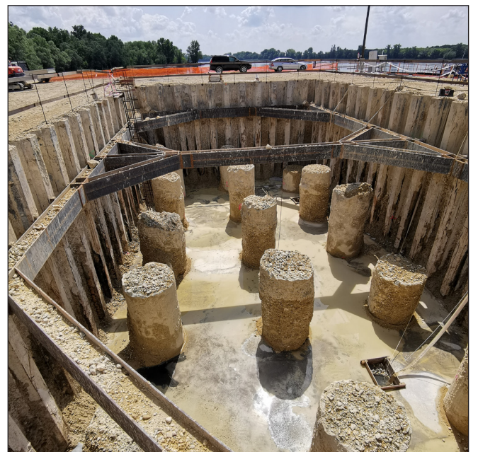
Fig 5: KP4 pier sheet pile cofferdam
