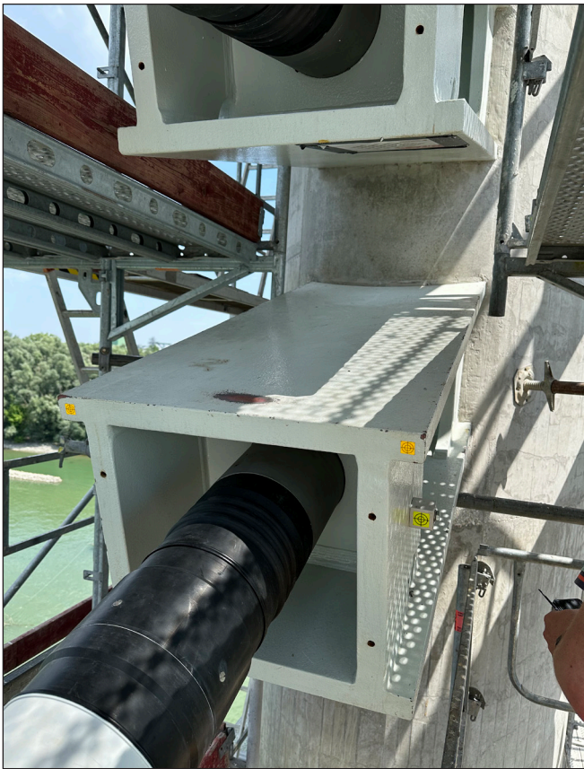
Fig 8: Upper anchorage node of the extradosed bridge
