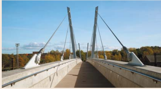
Fig. 4 View of completed pylons
