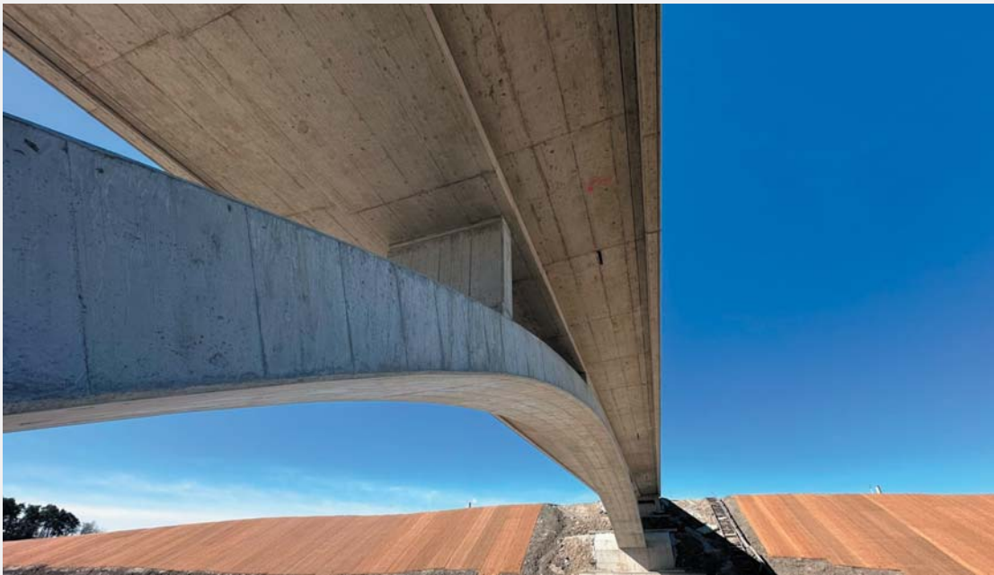
Fig. 6 Detail of the arch load-bearing structure of Bridge No. 212
