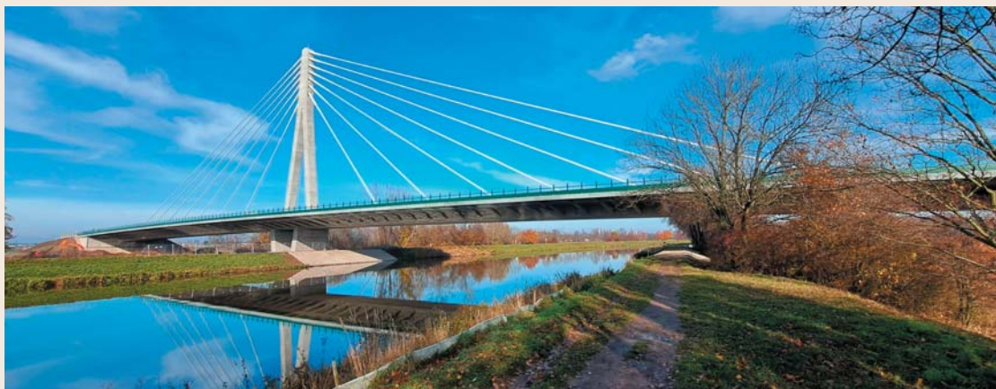
Fig. 1 Completed bridge Obr. 1 Dokončený most
