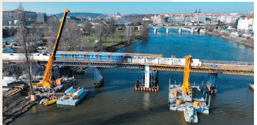
Fig. 10 Placing of a segment for the 4th stage from a pontoon
