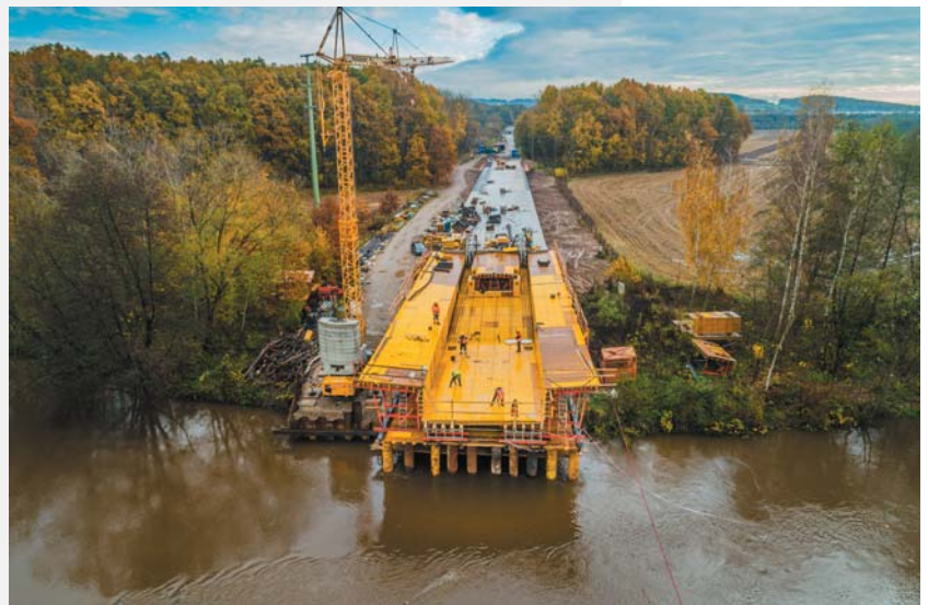
Fig. 5 Staged construction of the bridge
