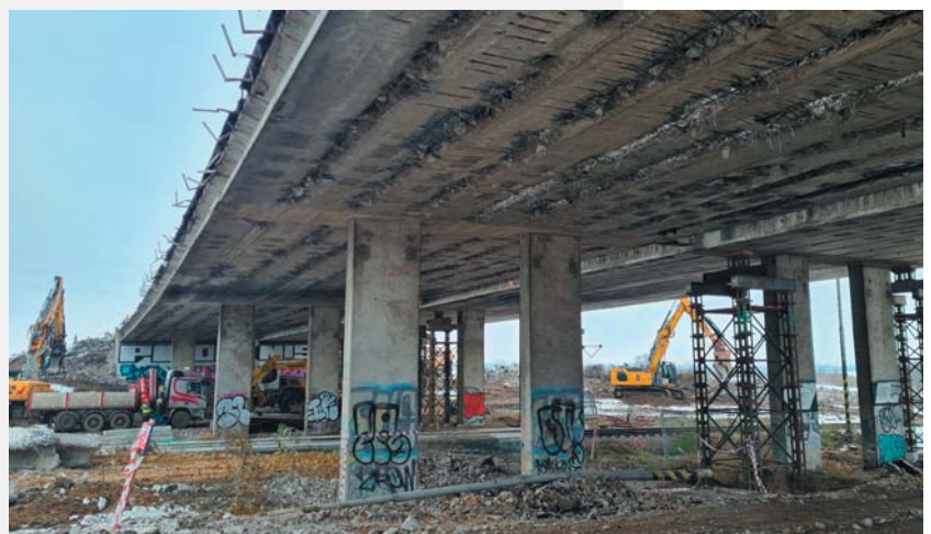
Fig. 5 Left bridge demolition
