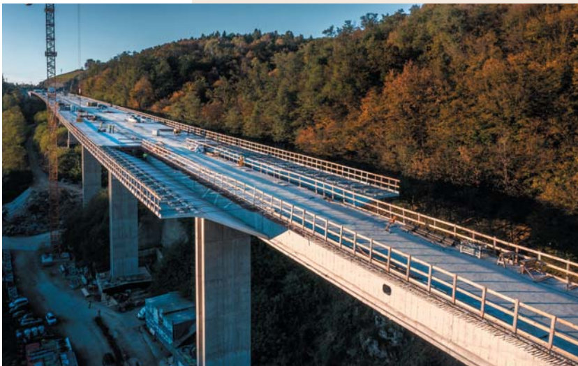
Fig. 18 Progressive construction of the deck
