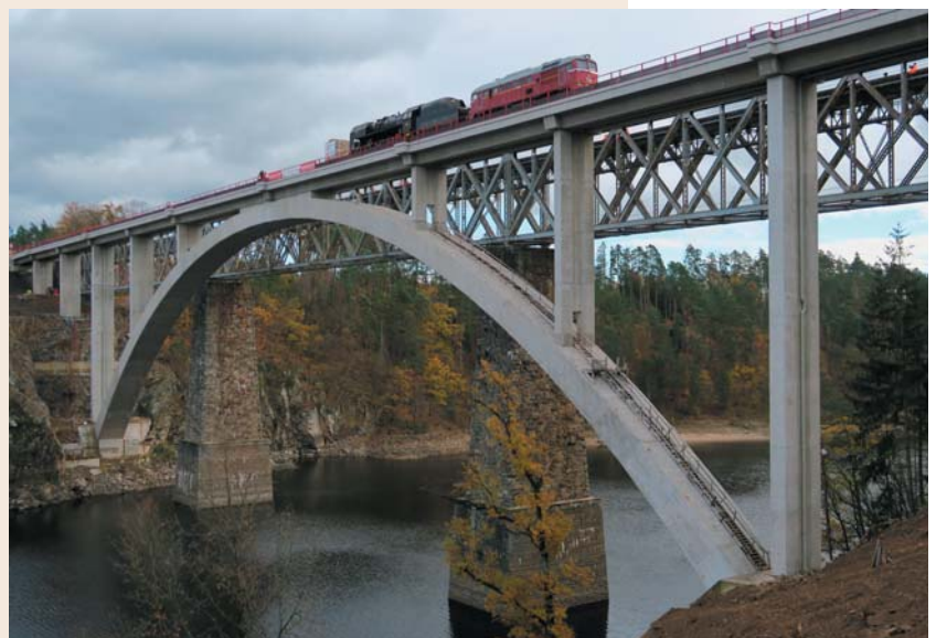
Fig. 10 Loading test of the completed bridge
