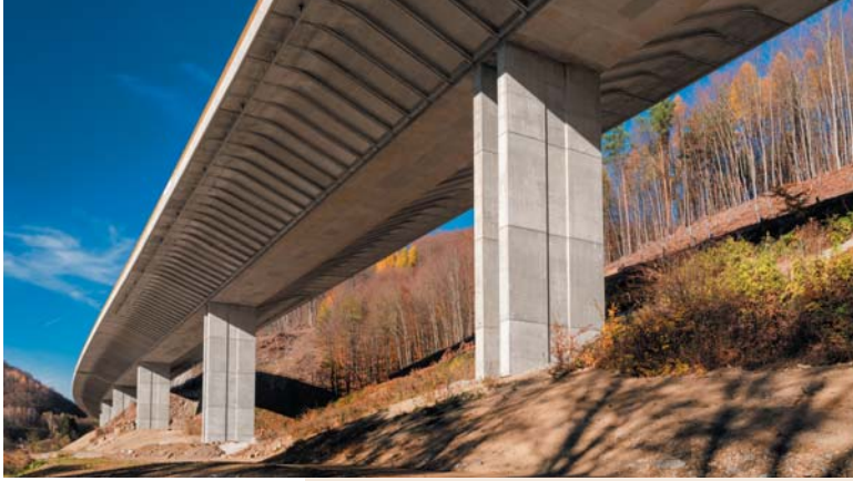
Fig. 15 Span-by-span constructed bridge
