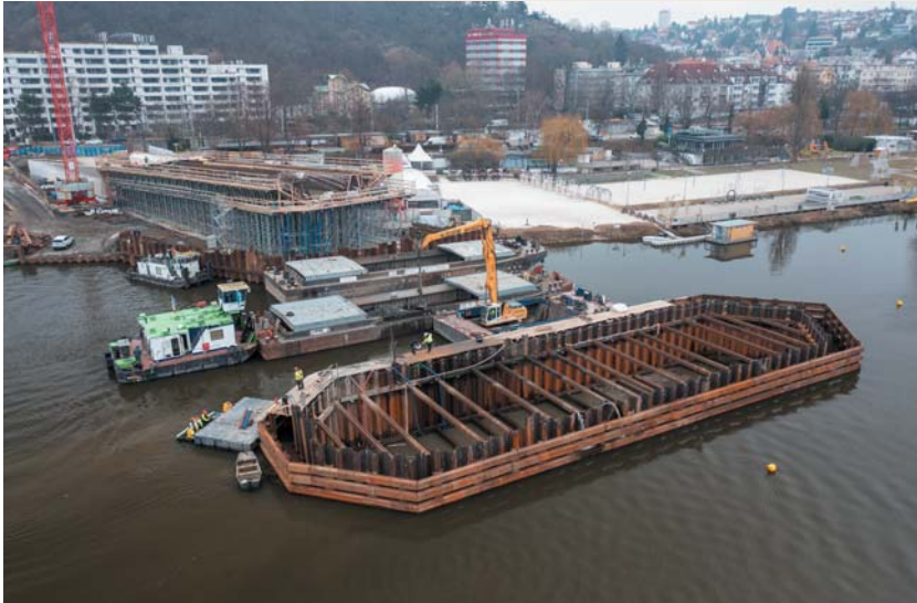
Fig. 5 Sealed cofferdam of pier P5
