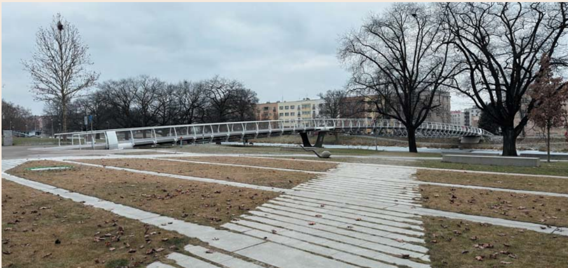
Fig. 7a, b Pedestrian Bridge over the Elbe River in Hradec Králové
