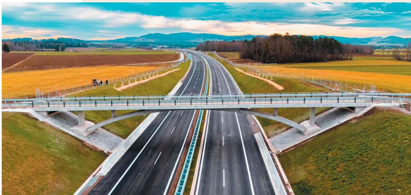
Fig. 5 Completed Bridge No. 212 before the opening for traffic
