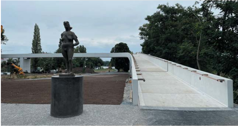
Fig. 19 Štvanice ramp with the "River" statue
