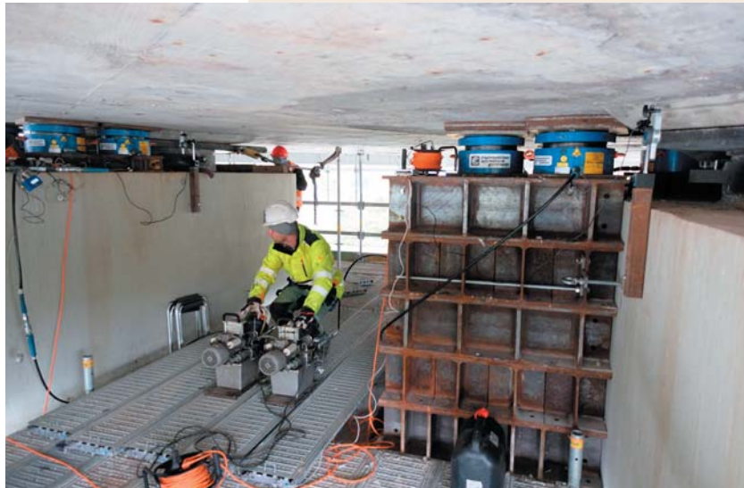
Fig. 8 Temporary supports of the bridge during the exchange of bearings
