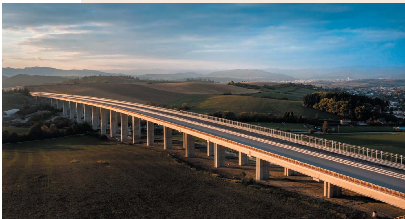
Fig. 1 Bridge 203 Obr. 1 Most 203
