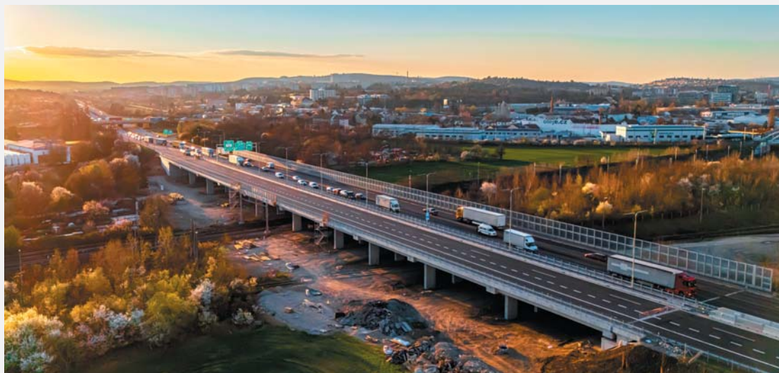
Fig. 10 Bridge before completion (source: MI Roads)
