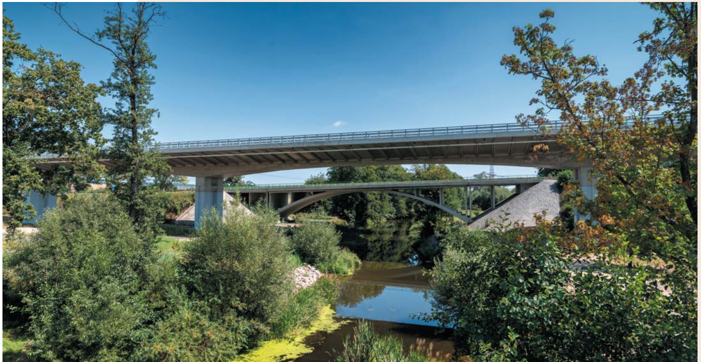
Fig. 1 Bridge over the Skalice River
