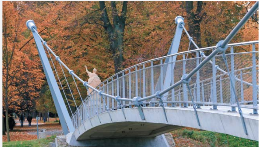
Fig. 9 Suspension cables and hangers
