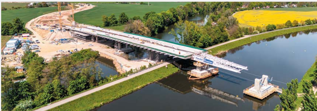
Fig. 4 Launching of the bridge deck
