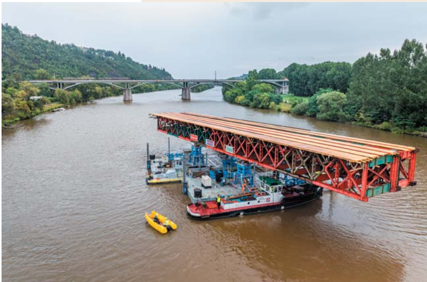
Fig. 13 Shaping of the superstructure
