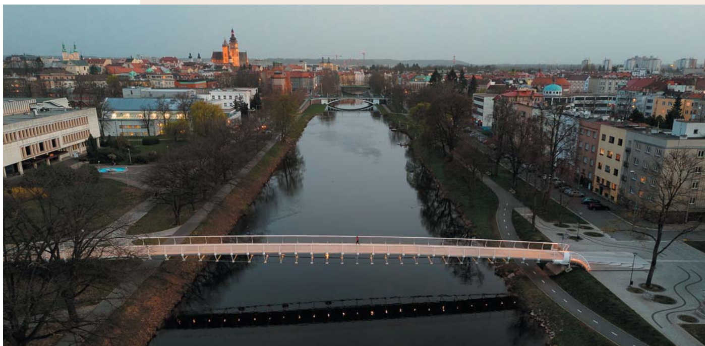
Fig. 1 Pedestrian Bridge over the Elbe River in Hradec Králové
