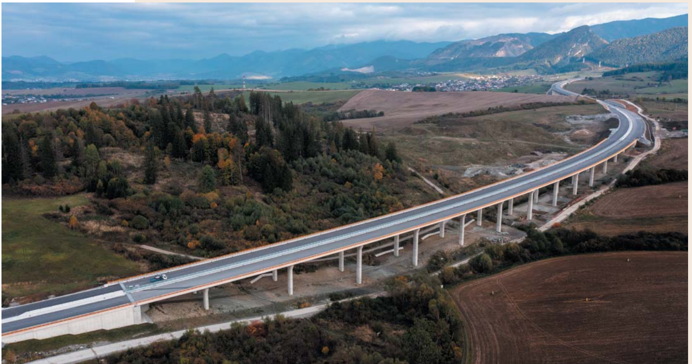
Fig. 1 Bridge 202 Obr. 1 Most 202
