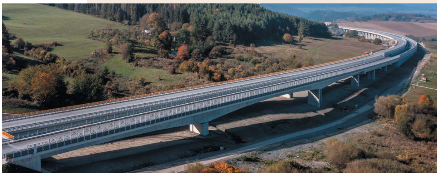
Fig. 1 Bridge 204 Obr. 1 Most 204
