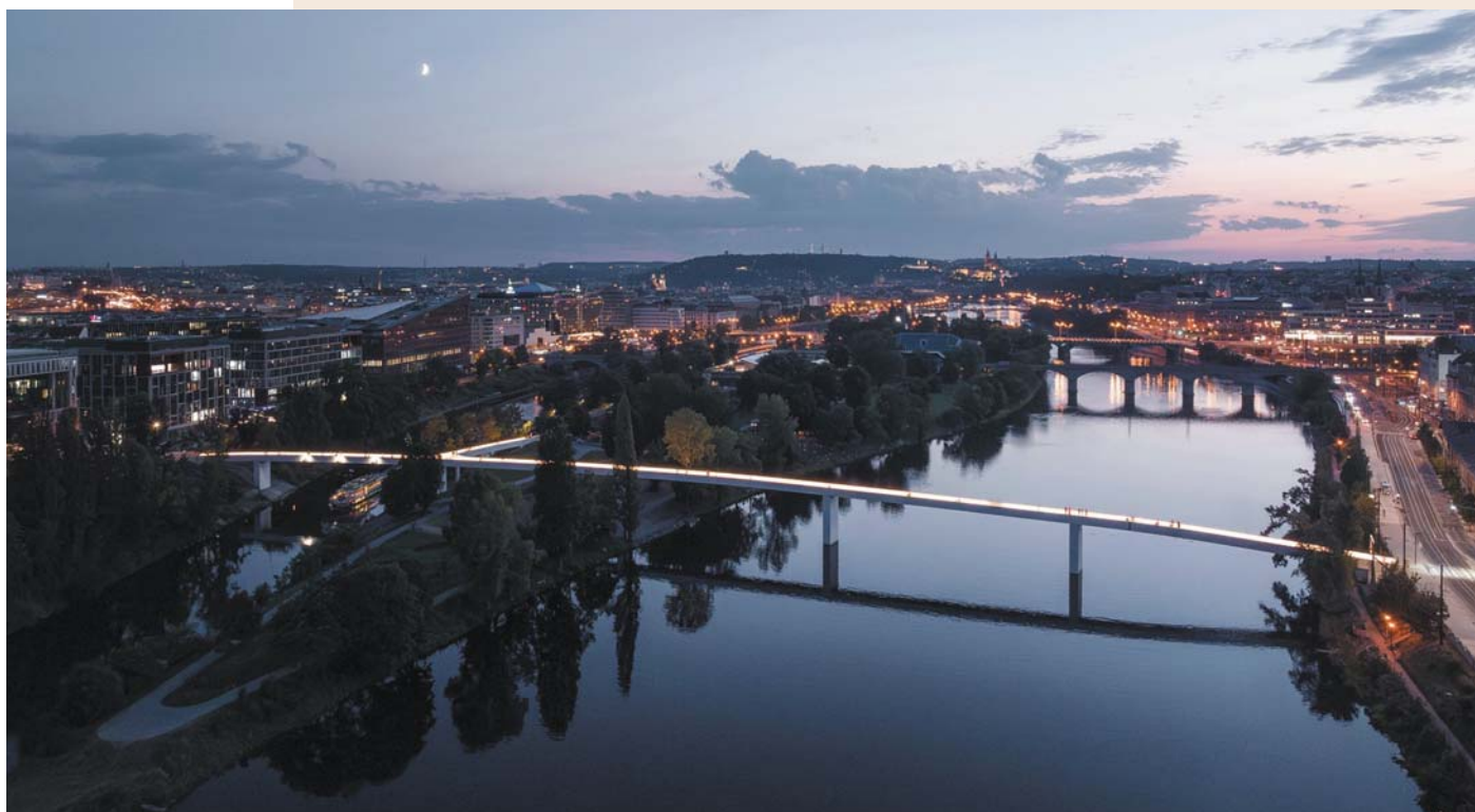
Fig. 1 The footbridge at dusk Obr. 1 Lávka za soumraku
