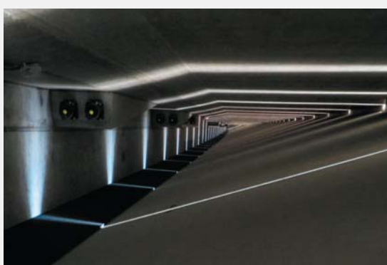
Fig. 9 View into the side chamber Obr. 9 Pohled do krajní komory
