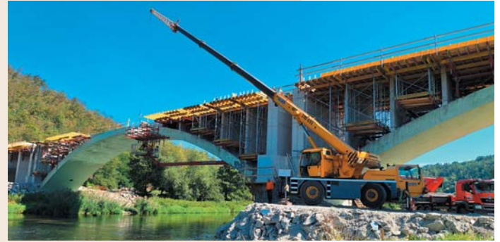
Fig. 2 Demolition of the bridge deck
