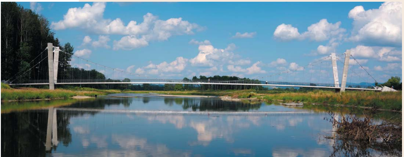
Fig. 1 Bridge across the Bečva River
