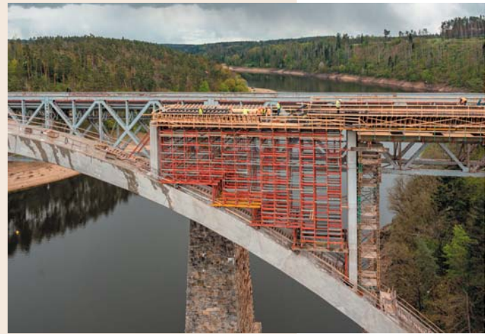
Fig. 8 Completed piers on the arch
