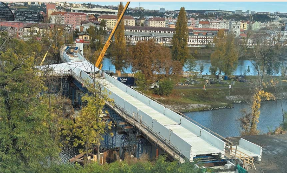
Fig. 12 Aerial view of the first 29 assembled segments
