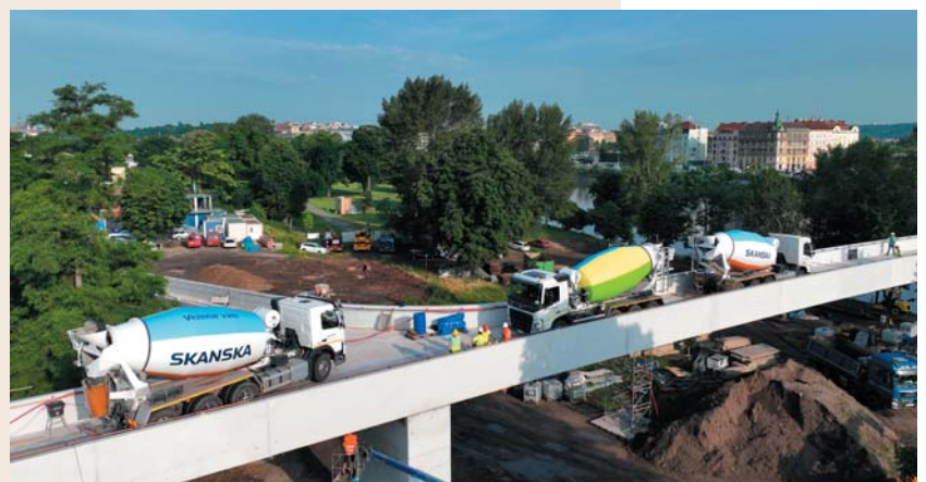
Fig. 18 Static load testing of the bridge
