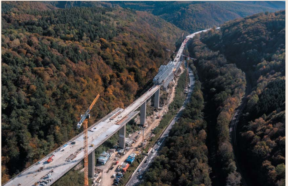
Fig. 15 Span-by-span constructed bridge
