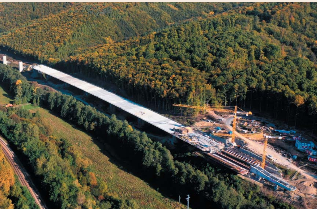
Fig. 19 Incrementally launched bridge
