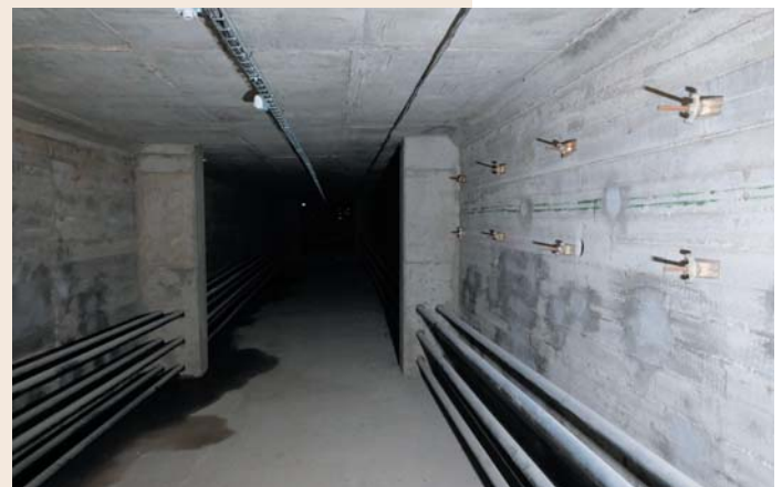
Fig. 6 External prestressing for strengthening of the superstructure
