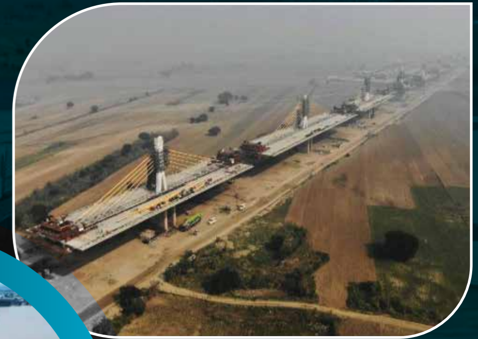
Extradosed Cable Bridge over river Ganga near Kacchi Dargah
