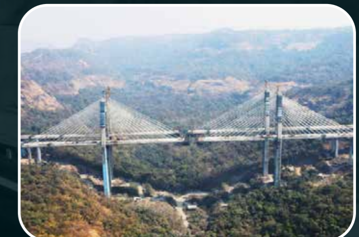
Viaduct 2 Under Construction
