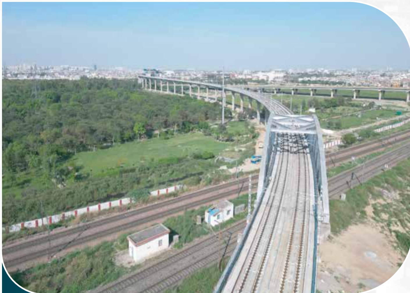
Completed Pre-Cast Slab Tracks on Viaduct
