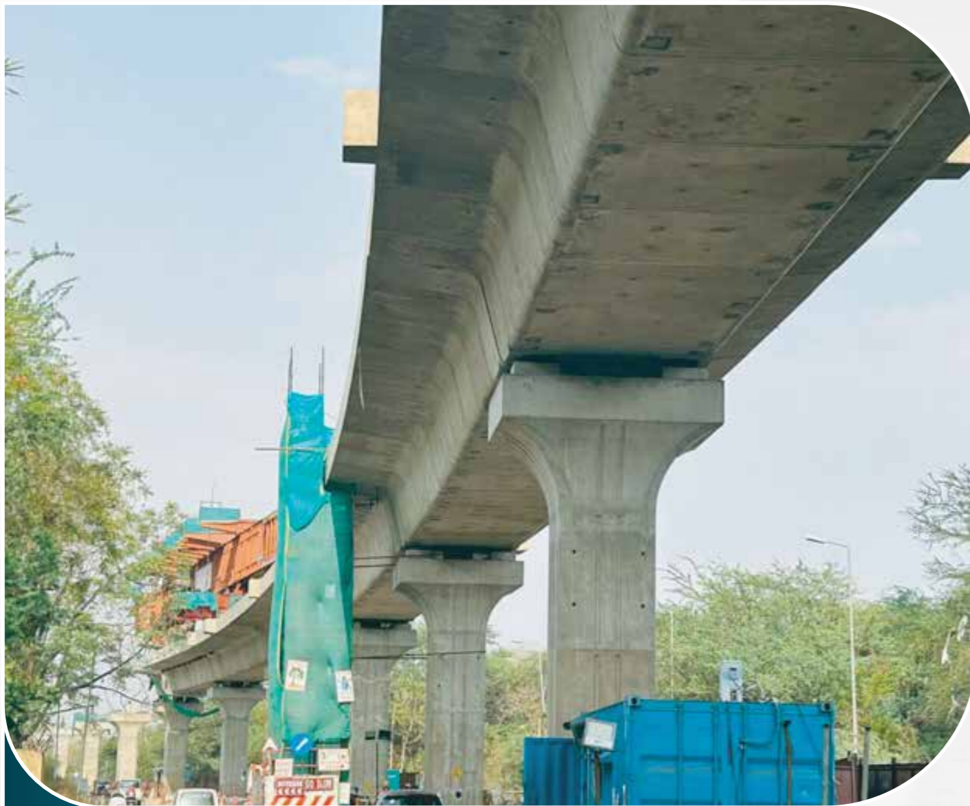
Metro Viaduct: Nagpur Metro
