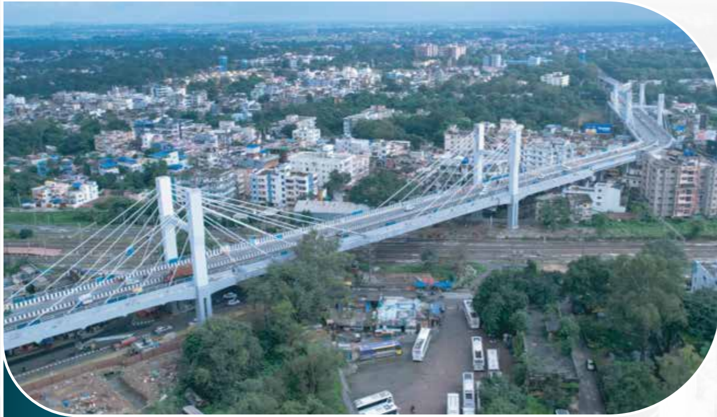
ROB Cable Stay bridge
