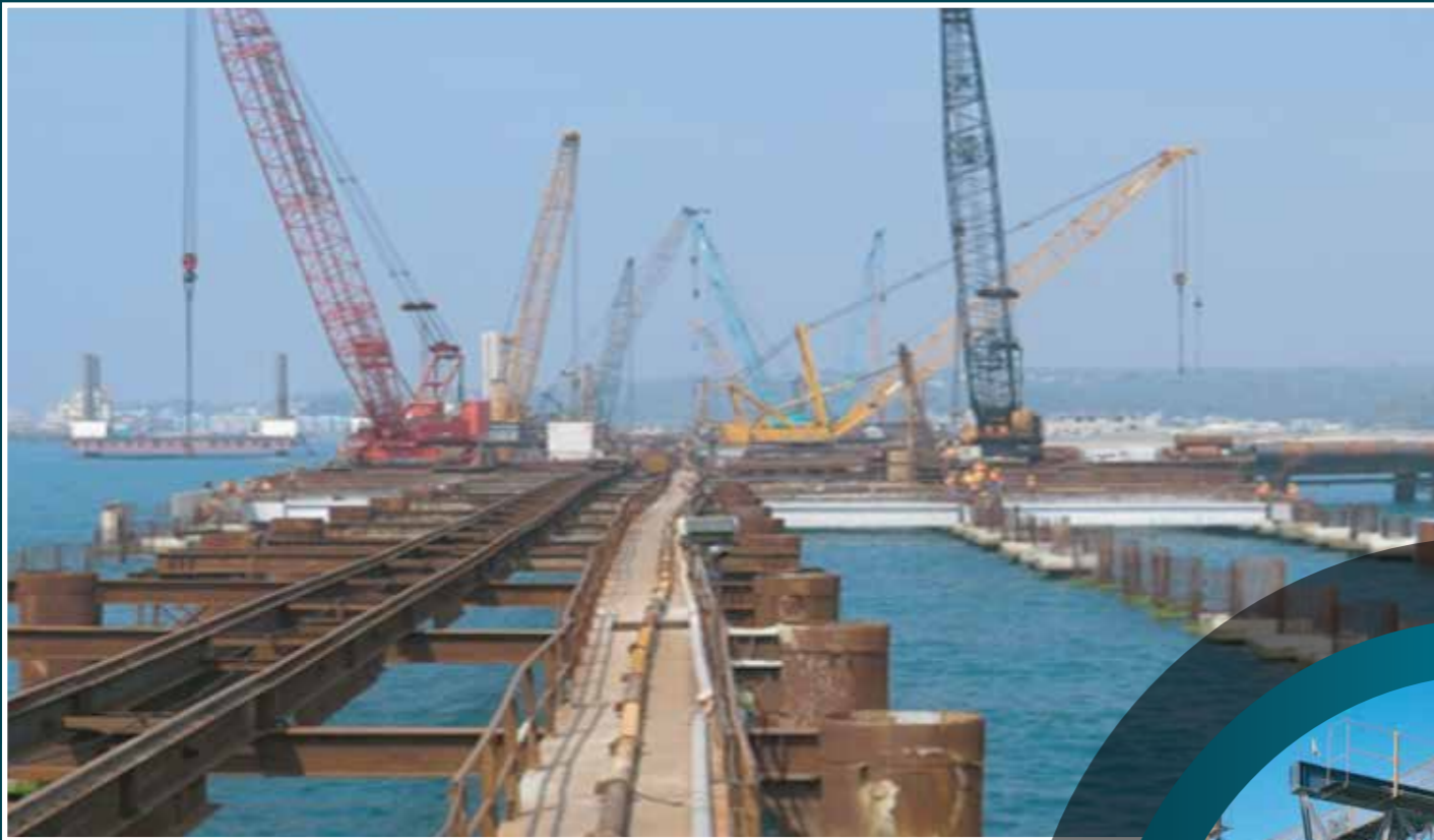
PILE CAP CONSTRUCTION
