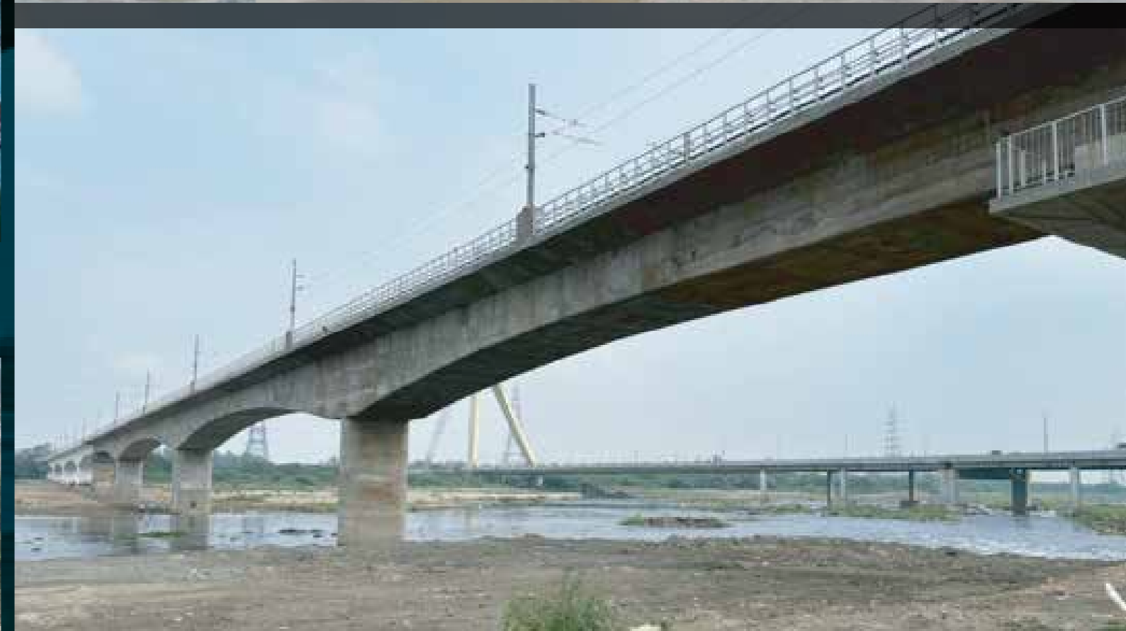
CLC over Yamuna – near Signature Bridge
