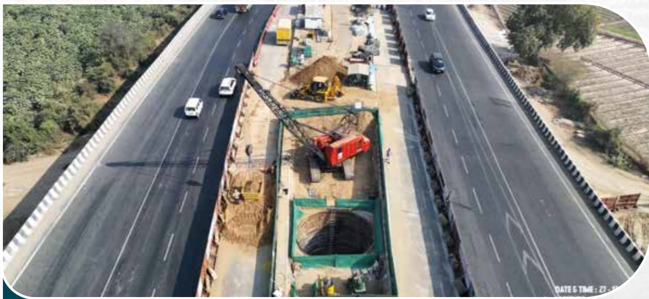
Shinso Pile Photograph
