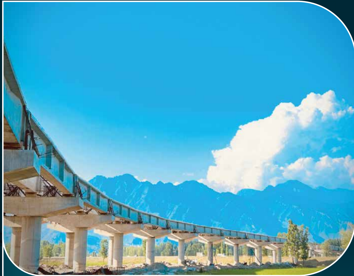
Interchange At Ch : 1+008
