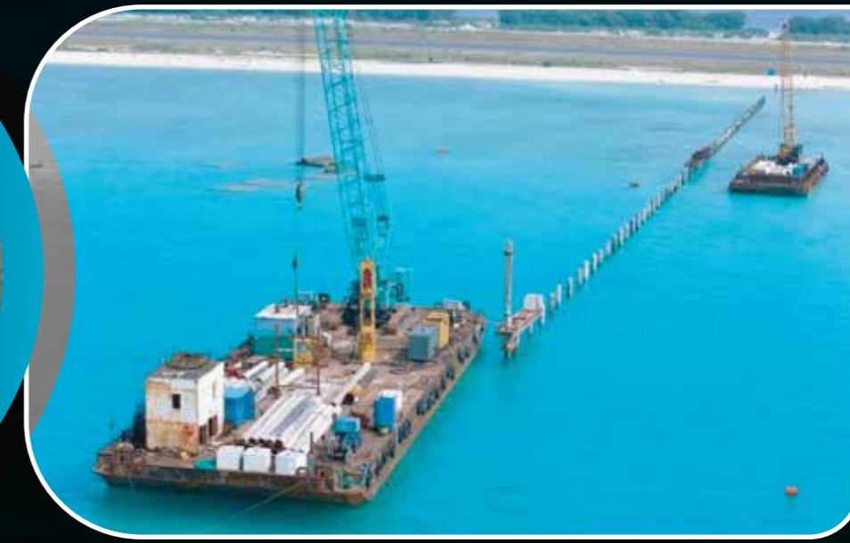
Spun Pile Driving.
