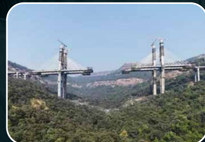
Viaduct 2 Under Construction
