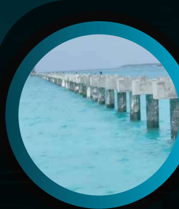
Casting of pile head.
