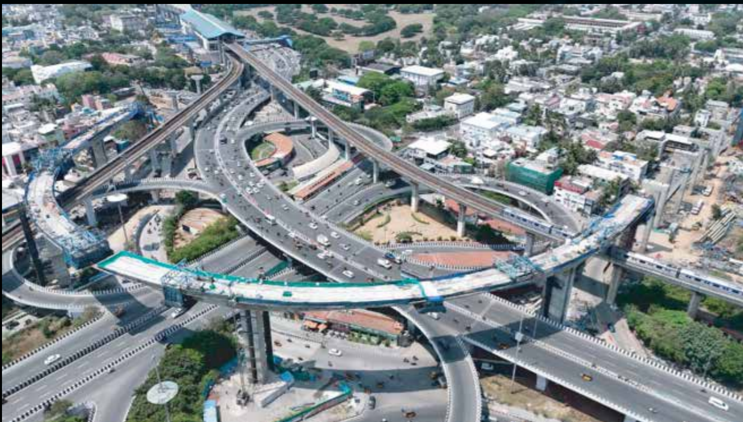
Construction of Curved Balance Cantilever Viaduct Spans
