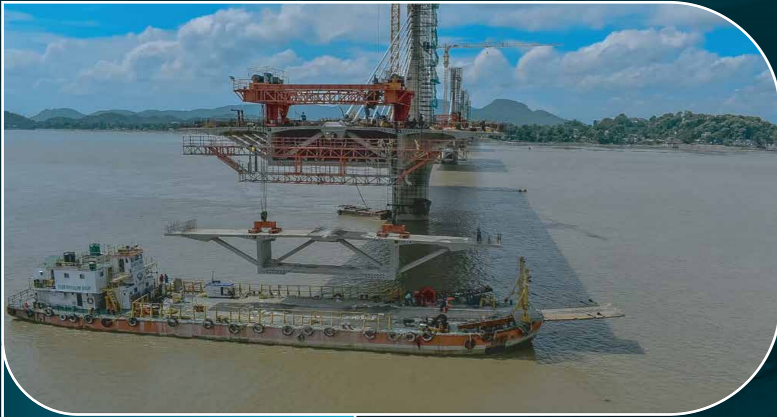
Segment Lifting above the Barge
