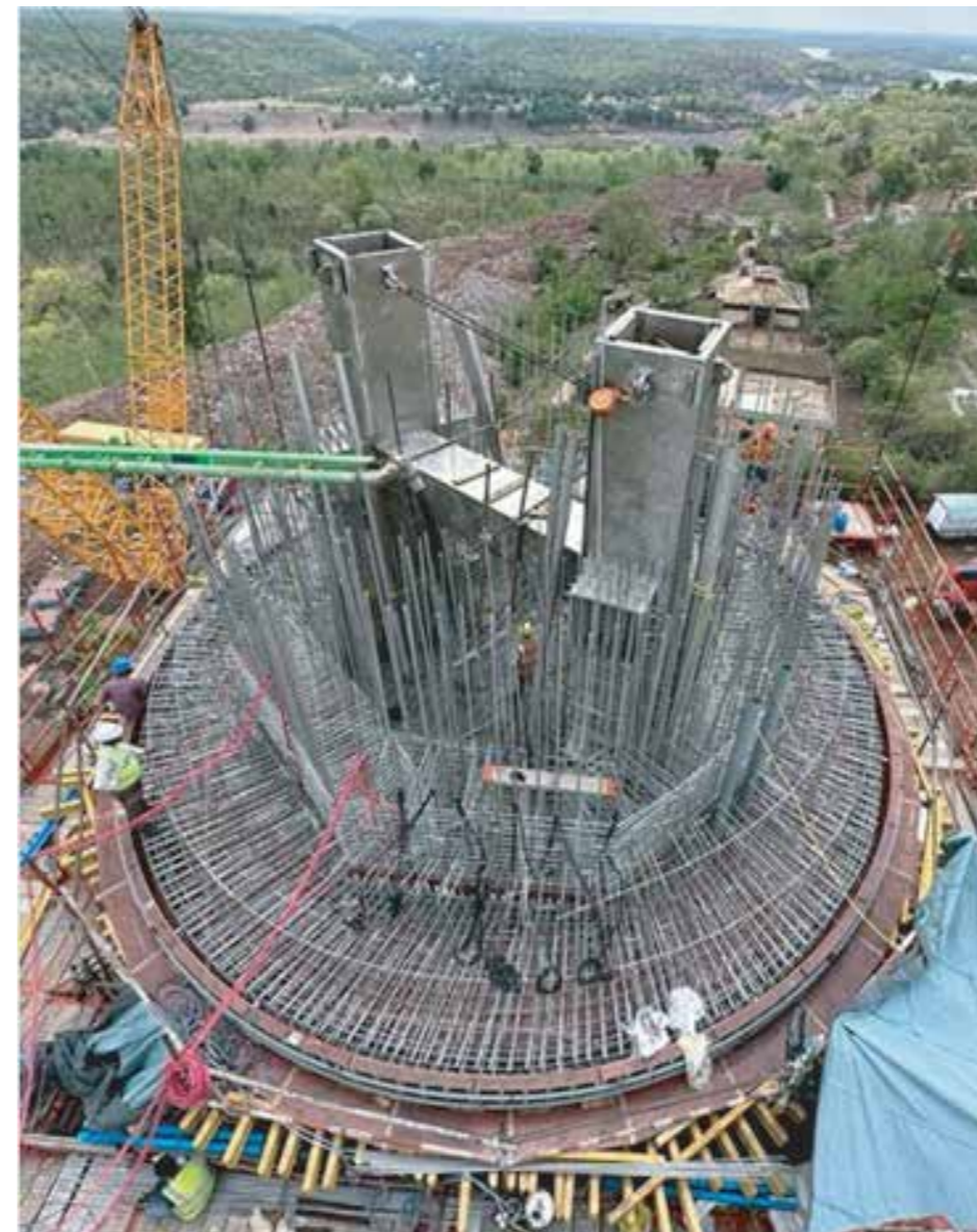
Structural steel Segment-1 Erection
