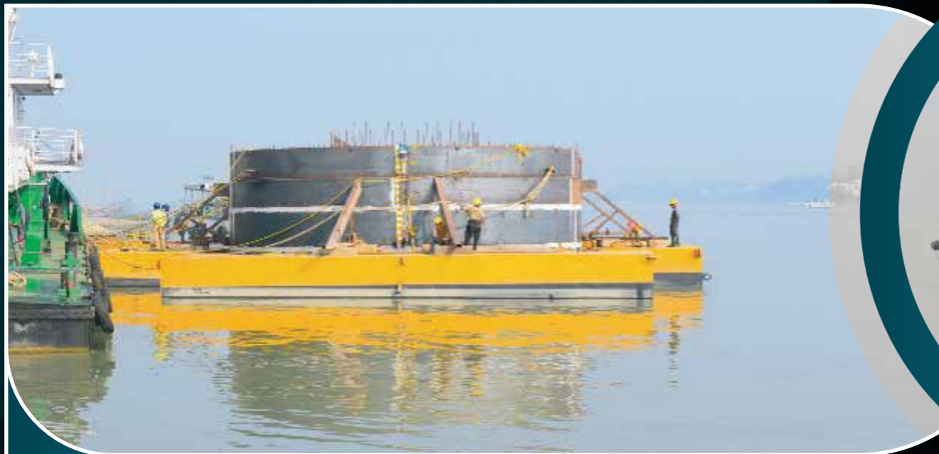
Towing the steel caisson on a barge
