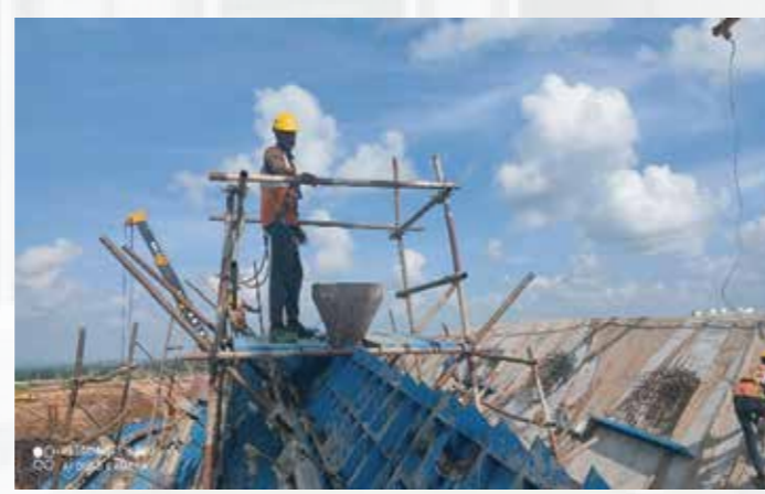
Concrete through Top Shutter
