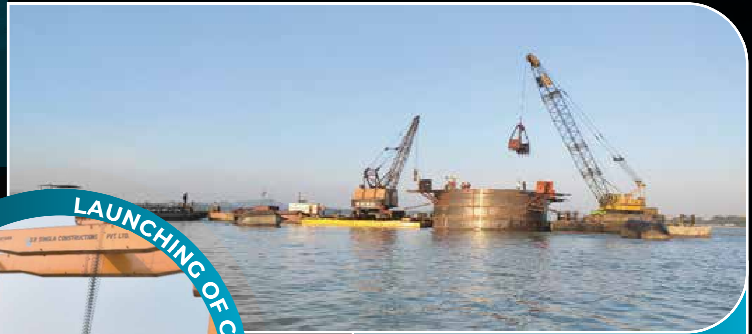
Caisson grounding at final location
