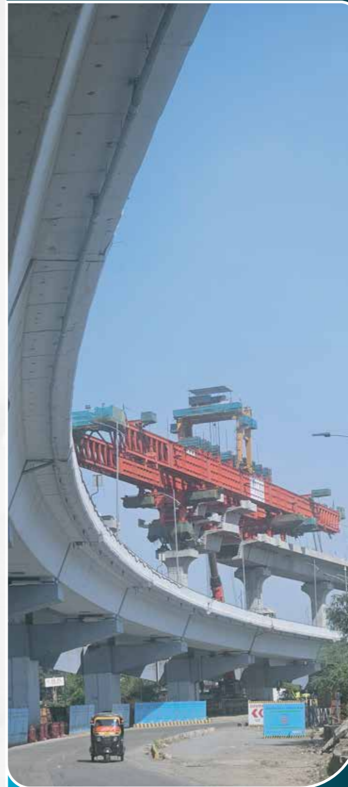
Double Decker Metro Viaduct : Nagpur Metro
