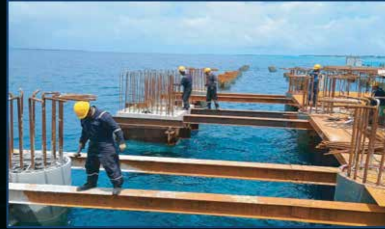
Erection of supporting arrangement. Bracket Fixing.
