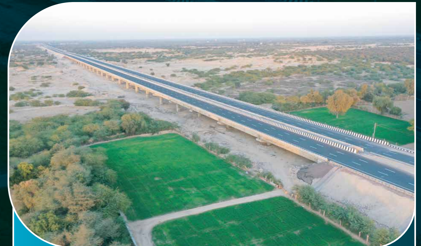
Lot-3 ; Package 3: Major Bridge (Ch. 64+420) on Luni River
