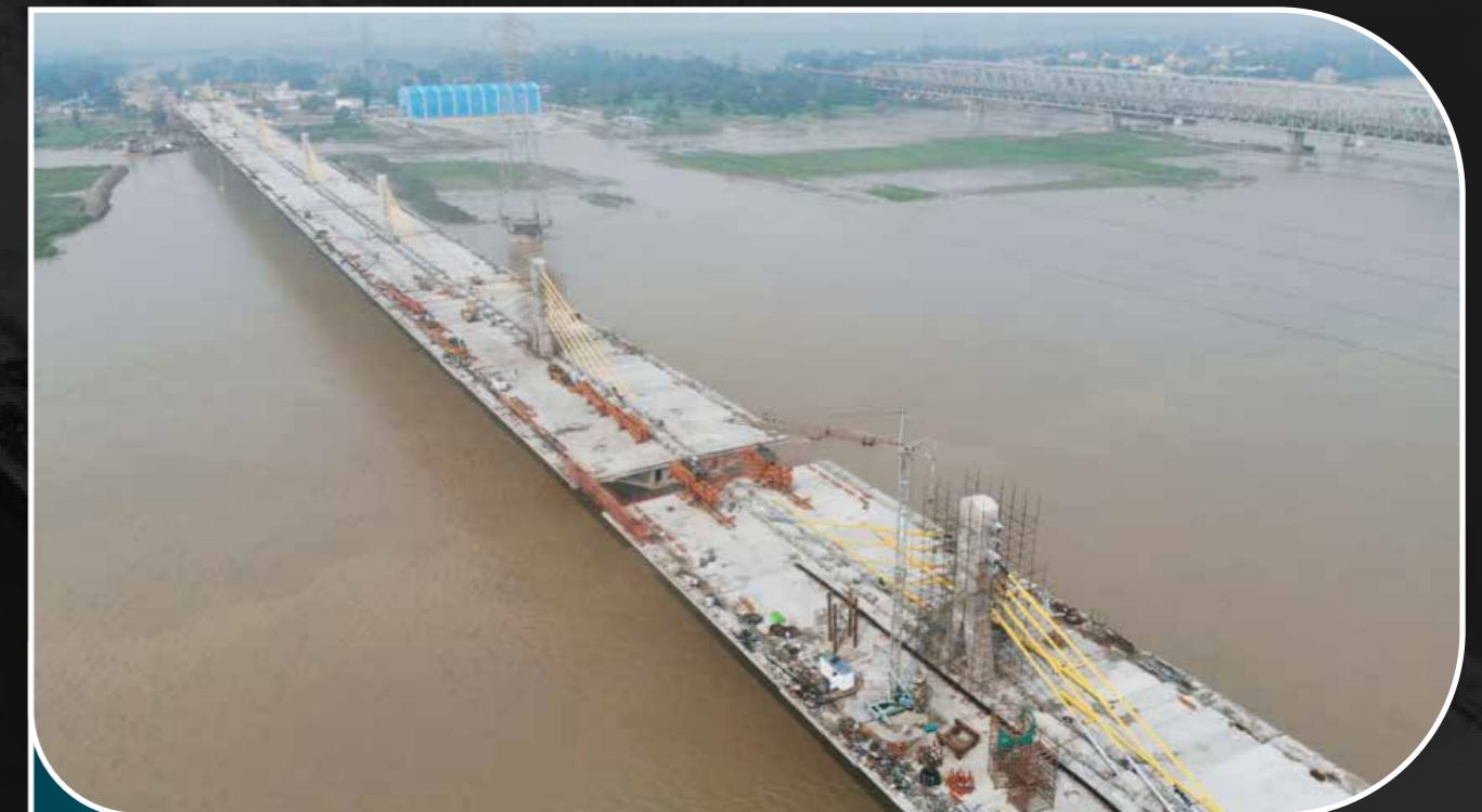
Superstructure under Construction
