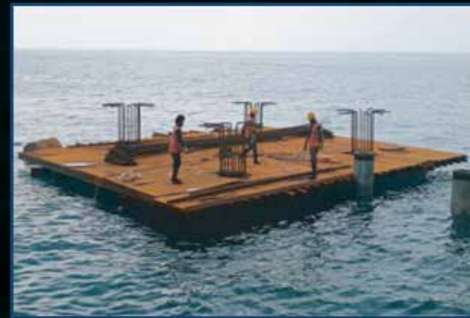
Erection Of Soffit shutter.
