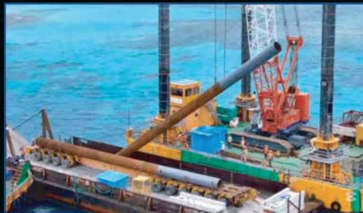
Liner Installation.
