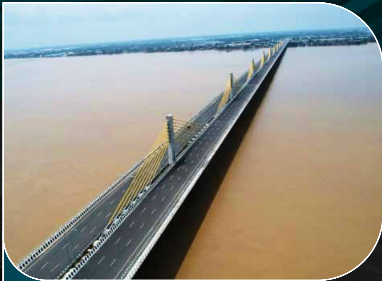
Extradosed Cable Bridge Over River Ganga Near Kacchi Dargah
