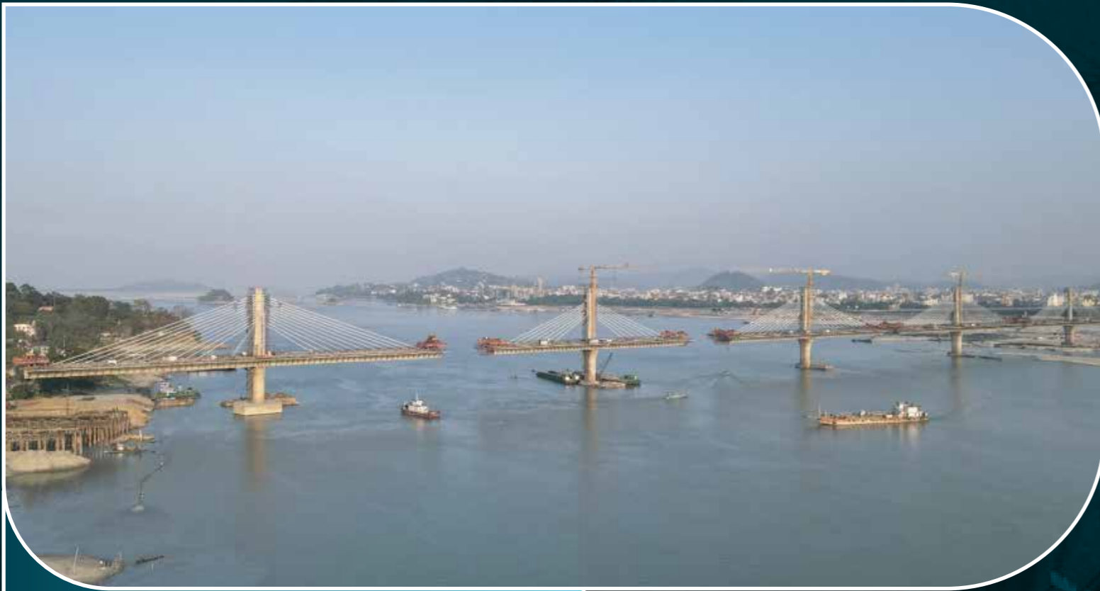
Superstructure construction in Progress
