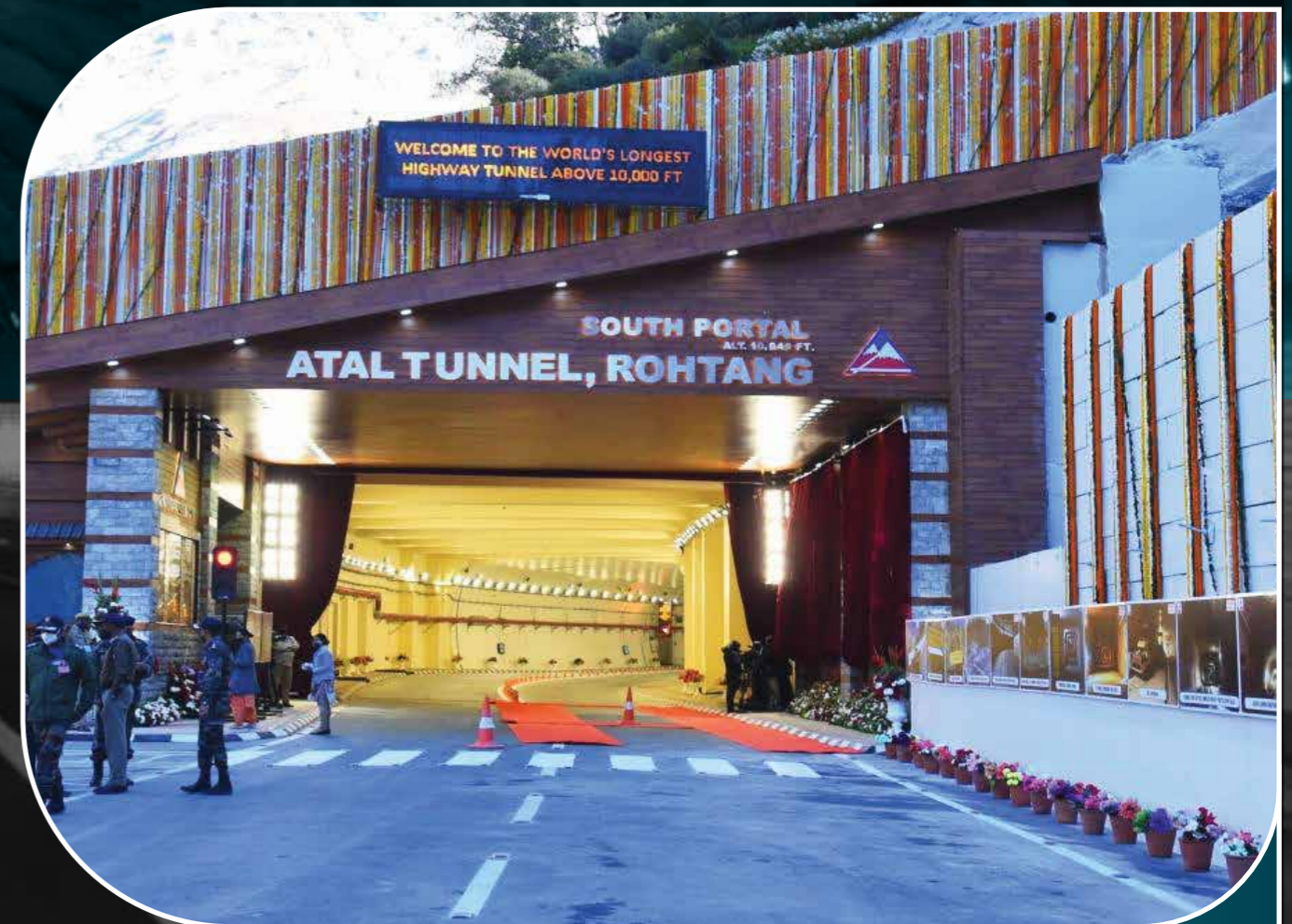
ENTRY TO ATAL TUNNEL FROM MANALI END
