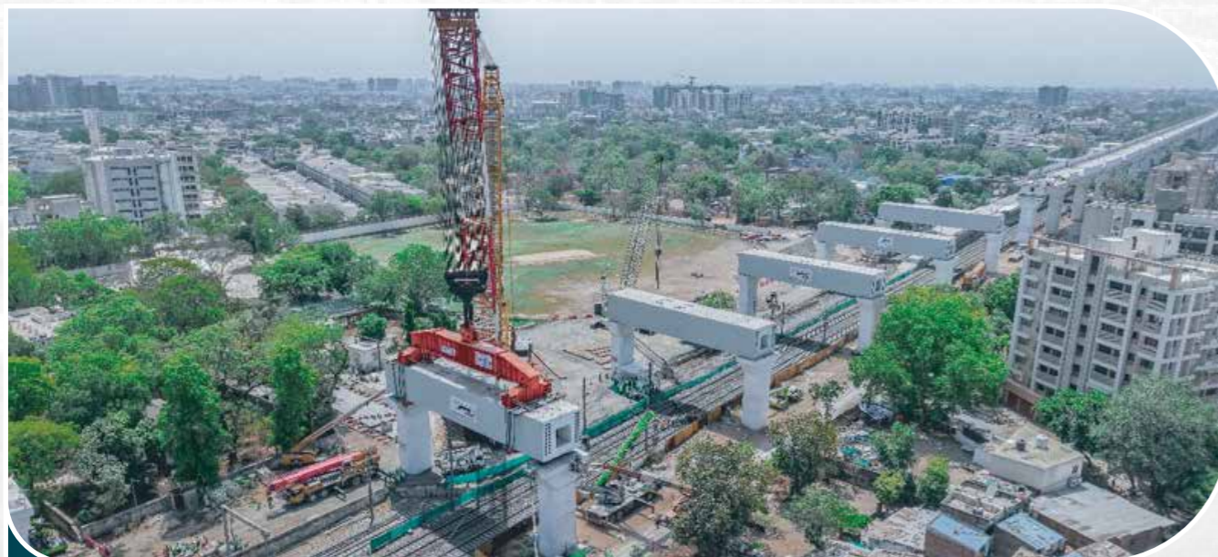
Shinso Pile Photograph
