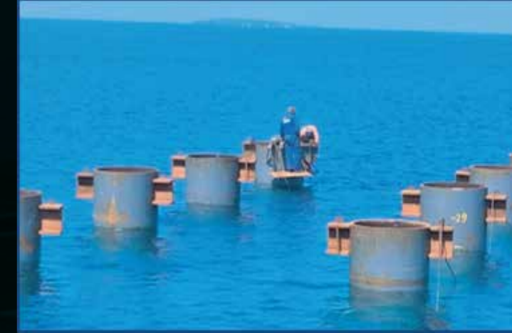
Erection of supporting arrangement. Bracket Fixing.
