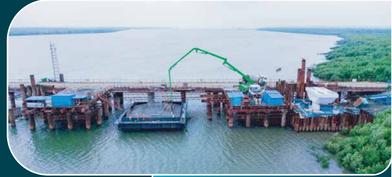
Vaitarna River Bridge (2.32KM long )
