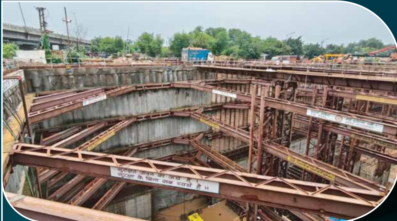
Temporary retaining system for UG Station
