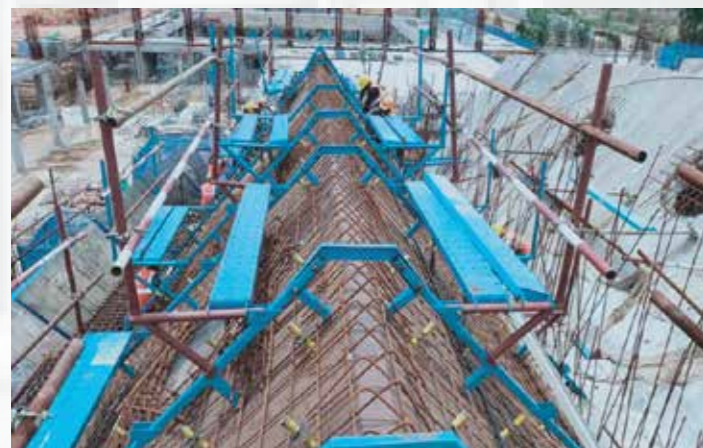
Rebar Tying Platform
