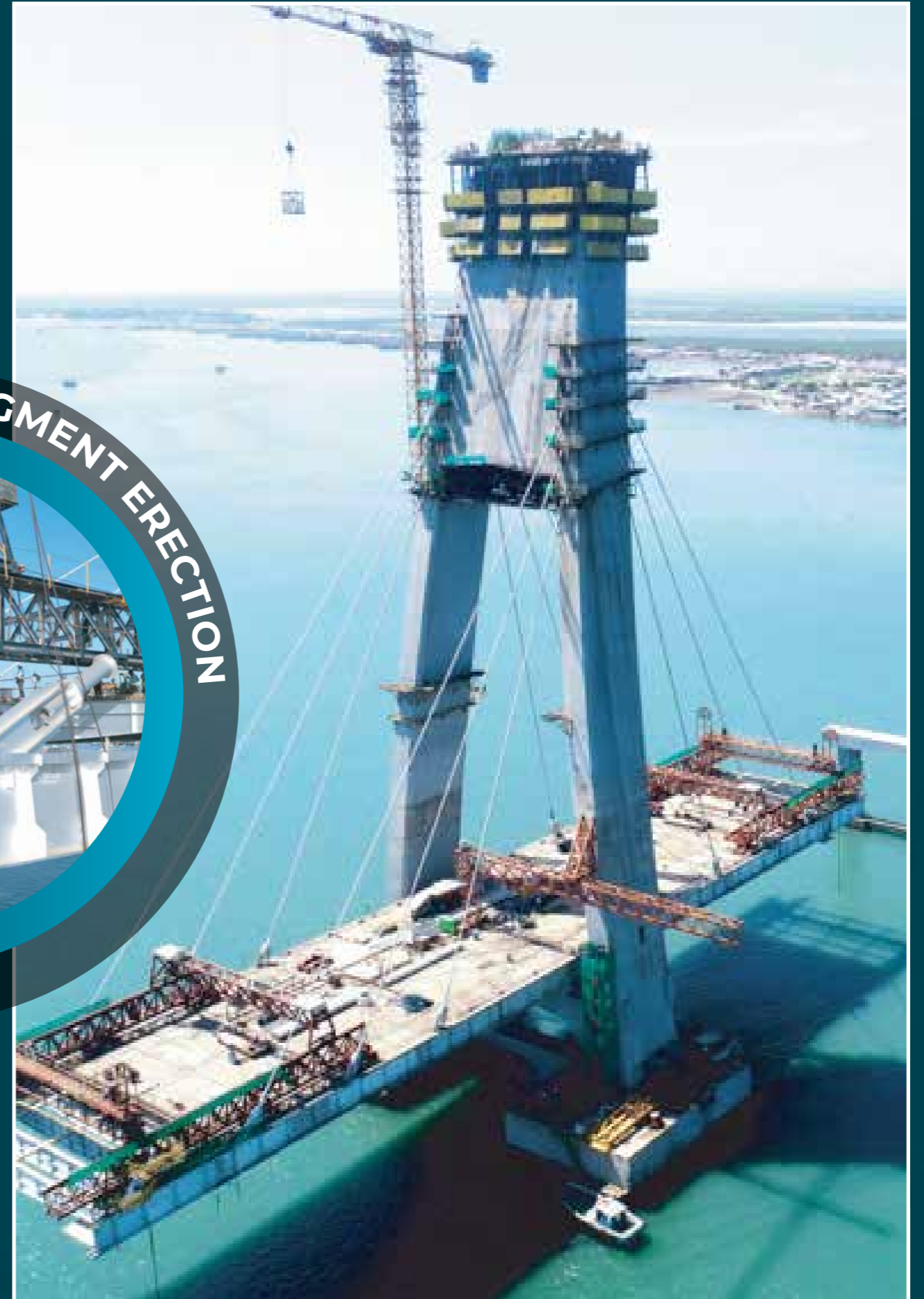
PYLON AND SUPERSTRUCTURE CONSTRUCTION
