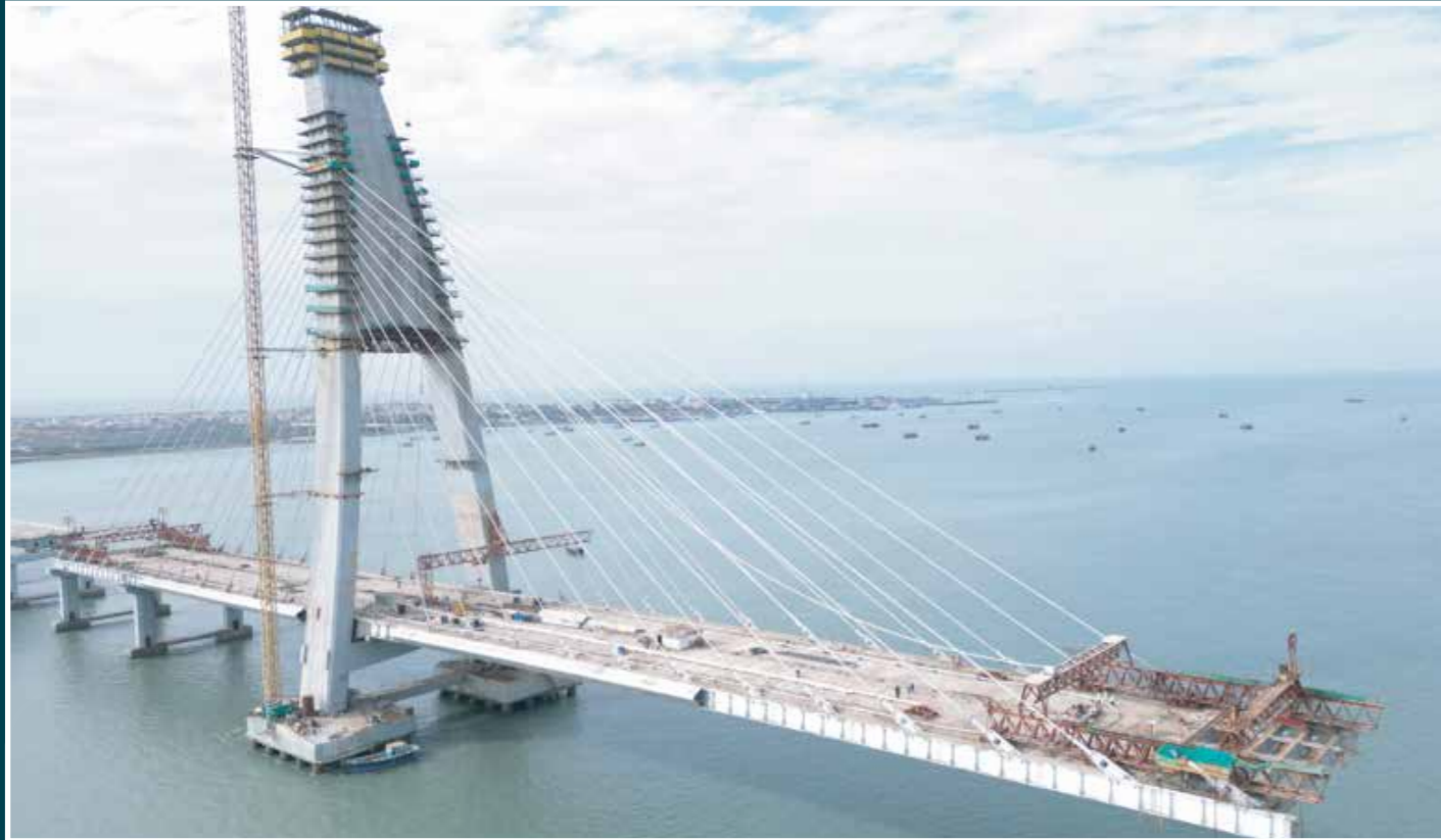
SUPERSTRUCTURE CONSTRUCTION
