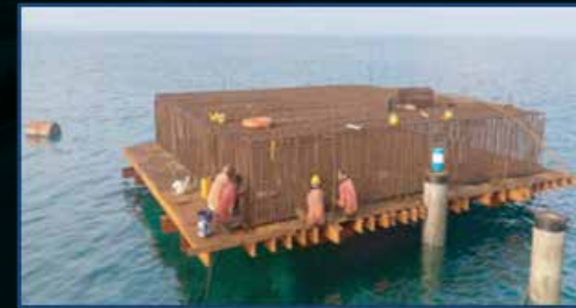
Fixing of Rebar.
