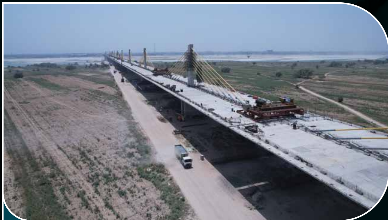
Extradosed Cable Bridge Over River Ganga Near Kacchi Dargah
