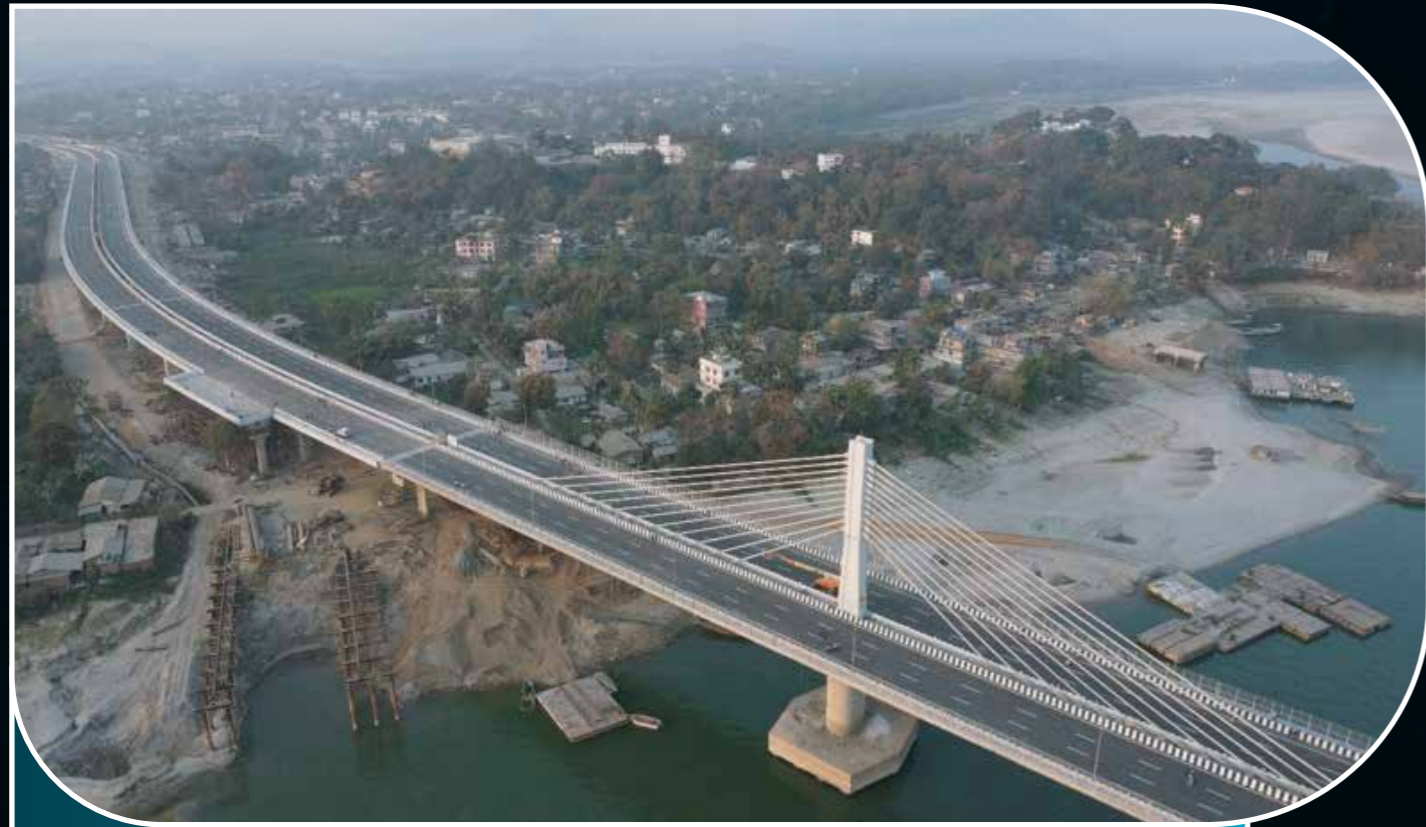
View of Completed Superstructure -North Guwahati side
