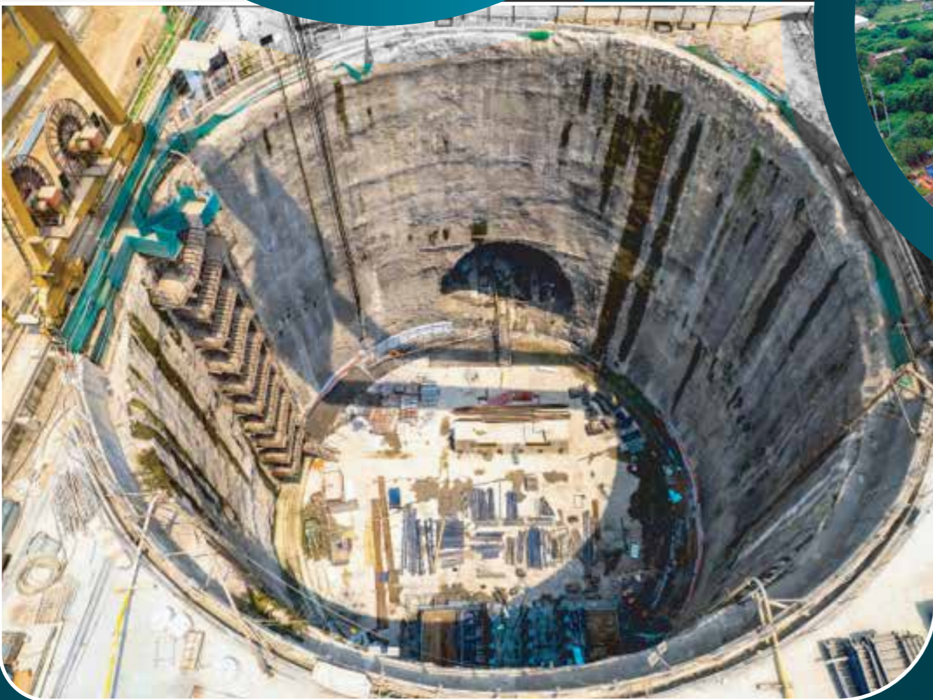
Work in Progress at Sawli Shaft, Ghansoli Maharashtra
