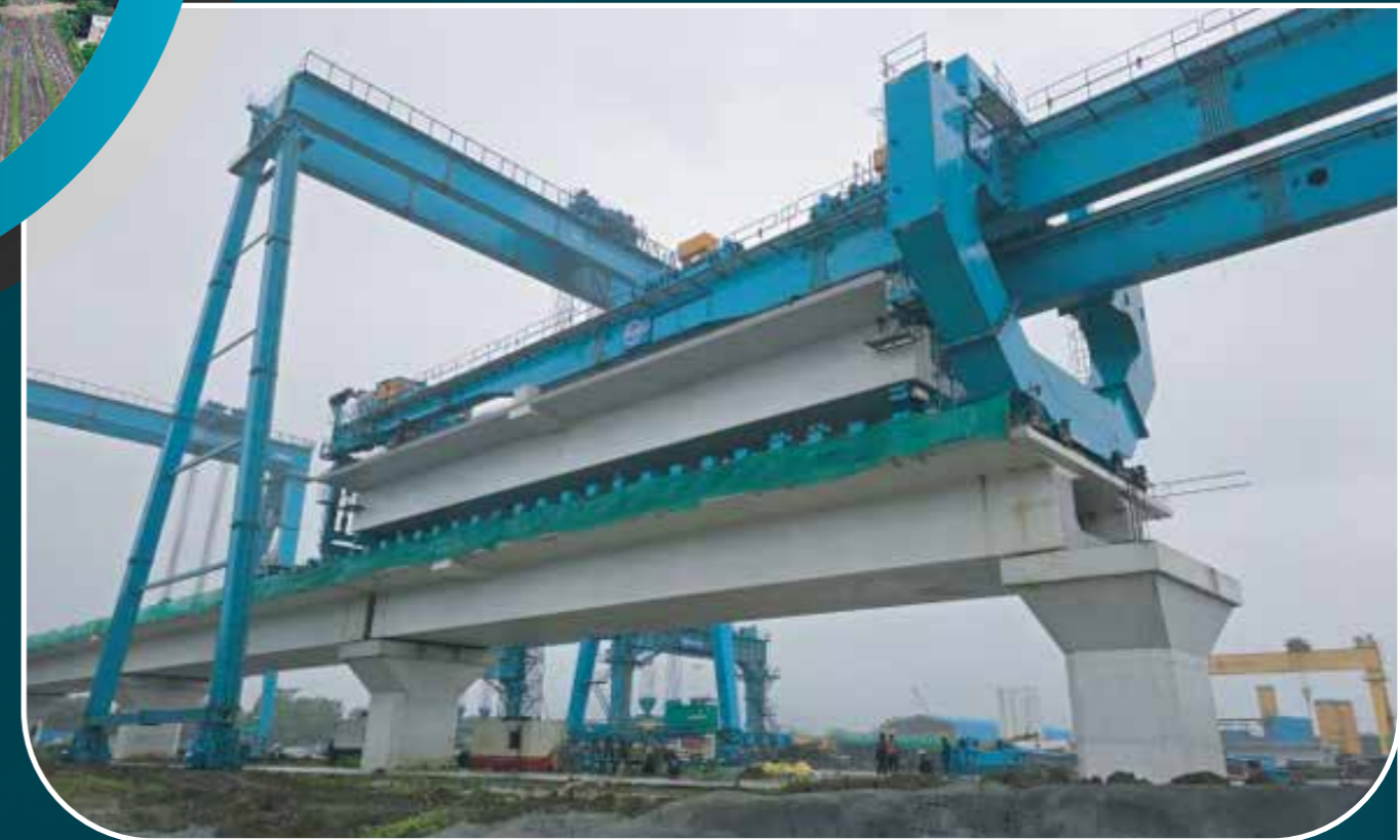
Work in Progress at Vikhroli Shaft, Maharashtra
