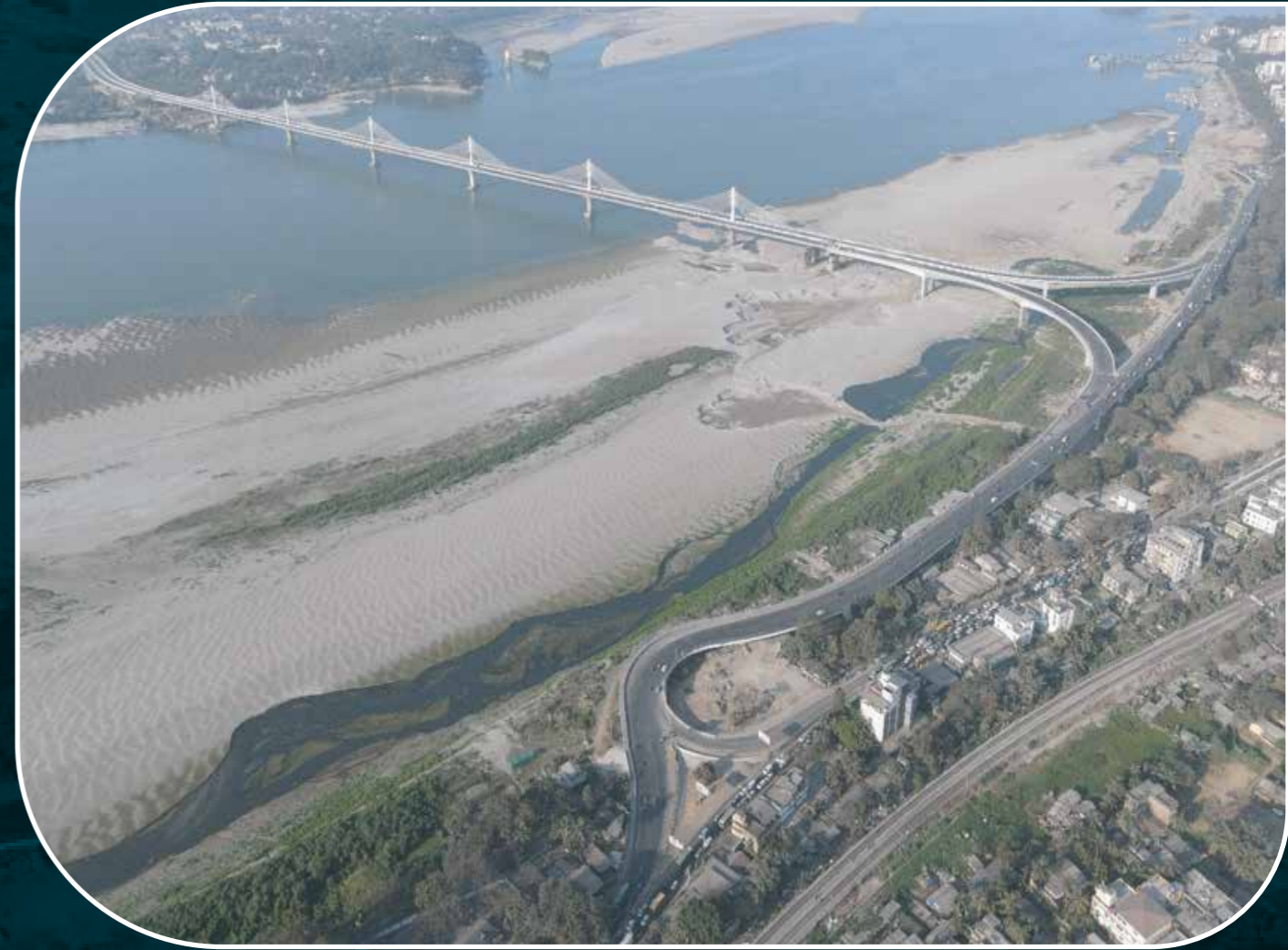
Overall view of the completed project
