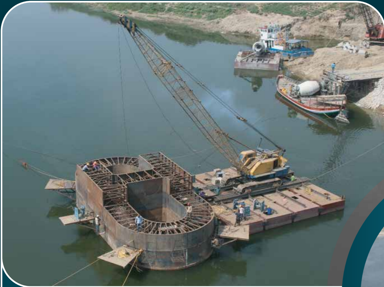
Foundation Under Construction
