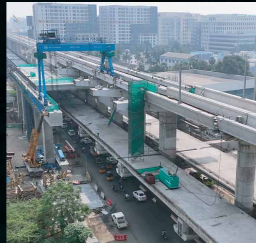
Erection of Station Precast elements with Double Decker Portion
