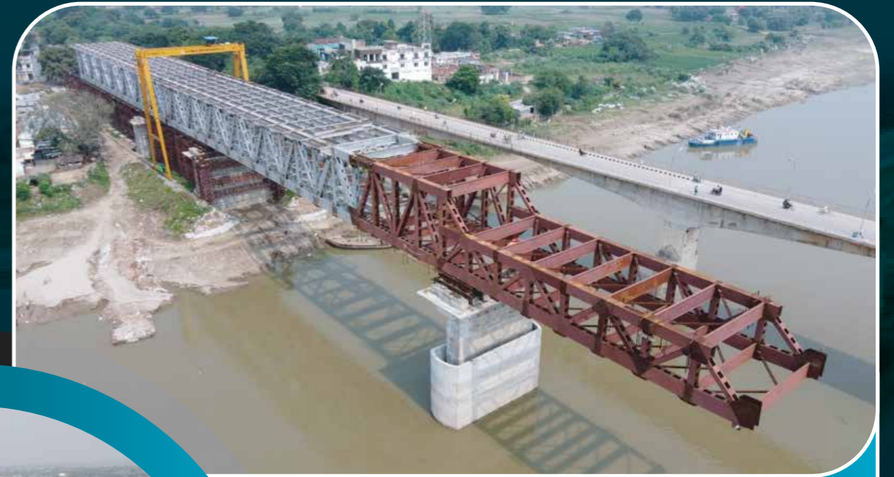
Superstructure Erection
