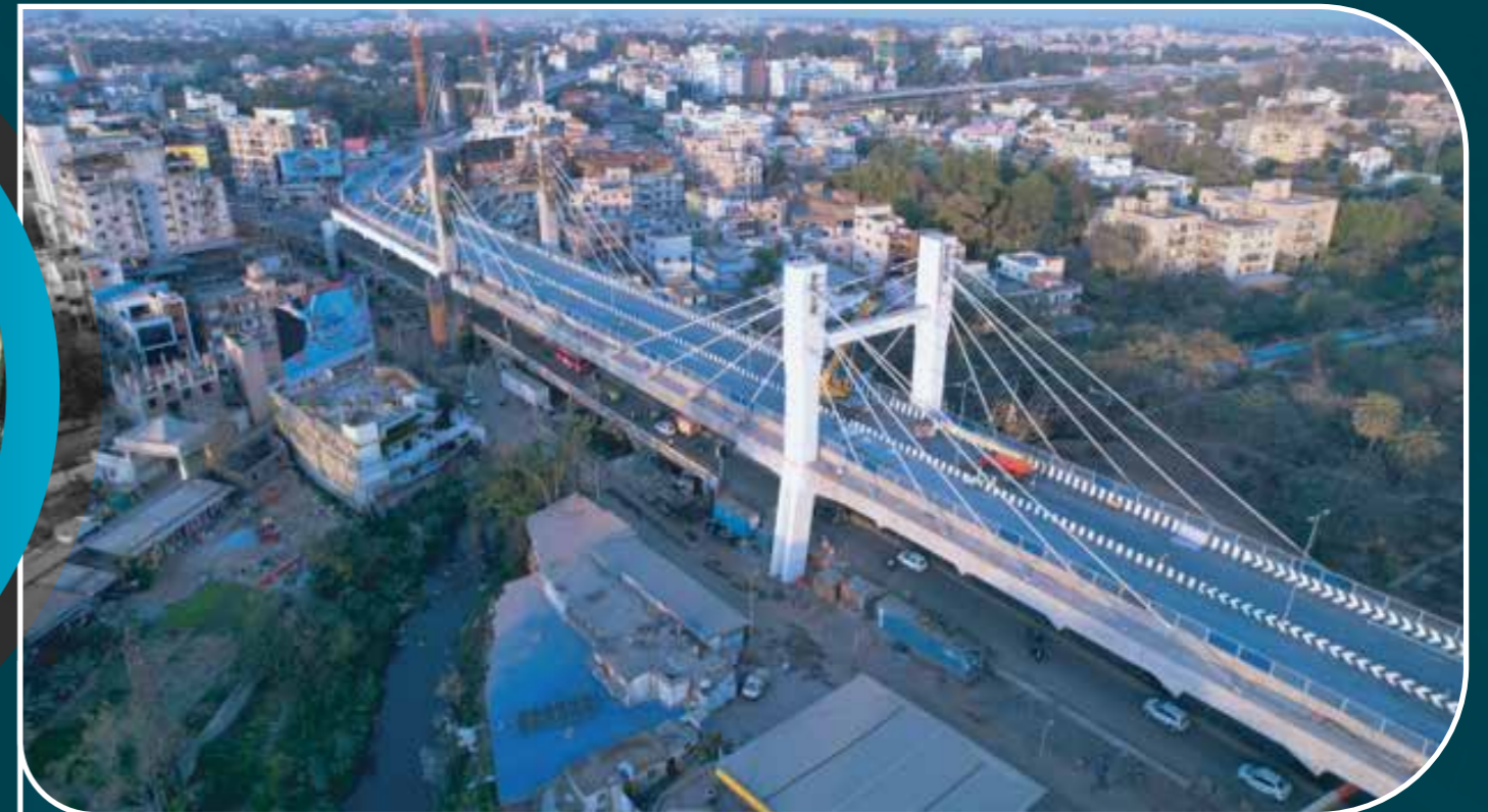
Harmu cable Stay bridge
