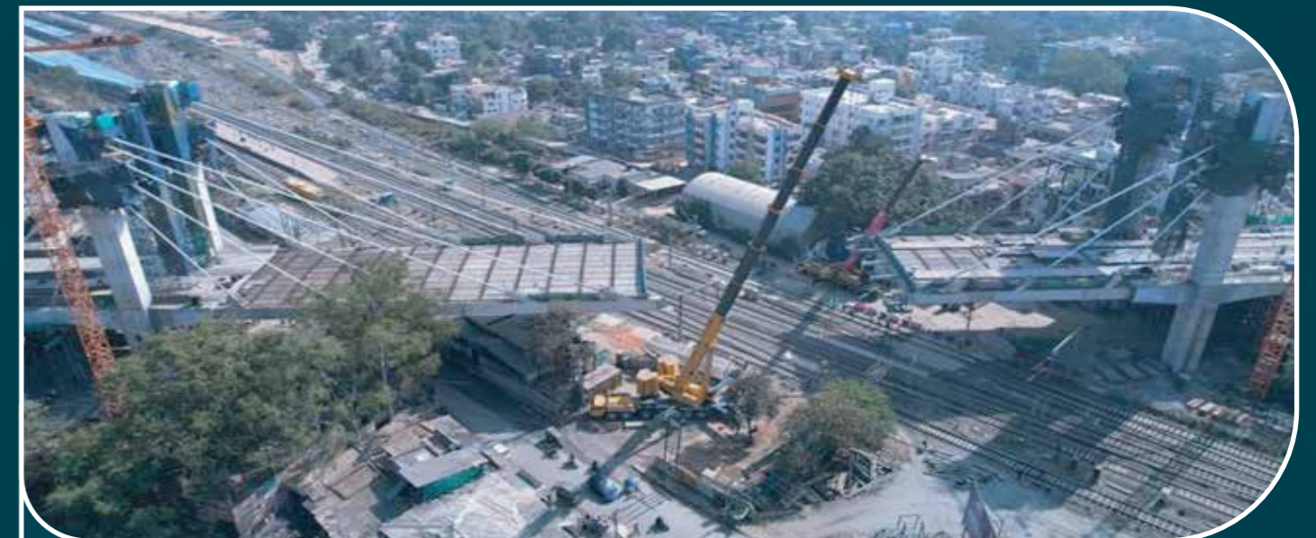
ROB Cable Stay Bridge Under Construction
