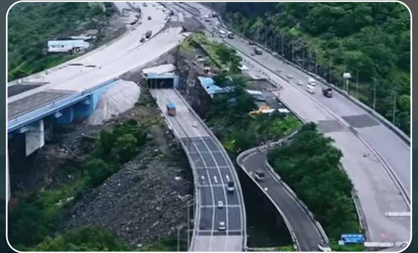
New Bridge on Slip road at Khopoli Exit and New VUP
