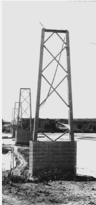
Bridge Towers over the Save River
