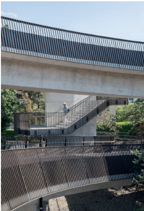
Fig. 8 Detailansicht Treppenturm. Detailed view of the stair tower. (© Beat Bühler)
