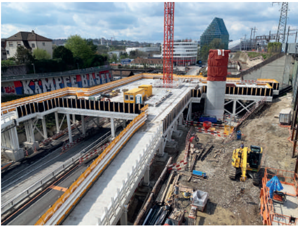
Fig. 5 Installationsplattform. Working platform.
