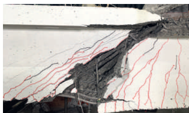
Shear failure in the beam web.
