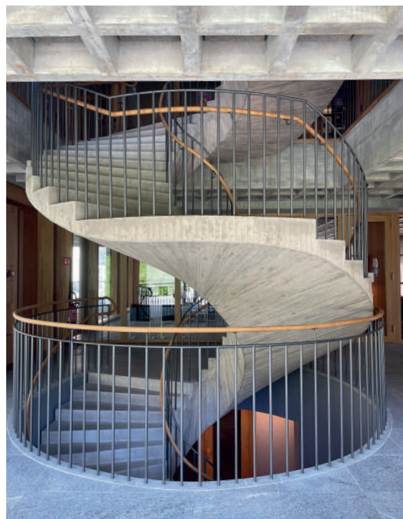
Fig. 10 La scala al pianterreno. The staircase on the ground floor.
