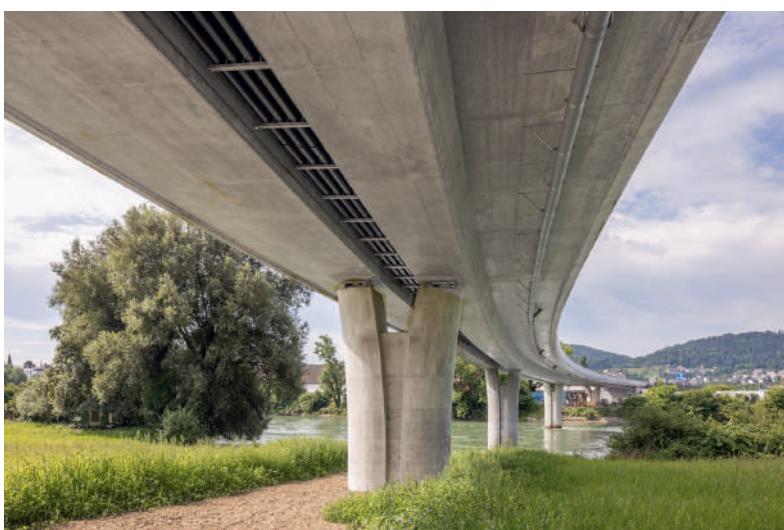
Fig. 5 Neue Reussbrücke, Blick von Norden Richtung Reuss. New Reuss bridge, view from the north towards the Reuss.
