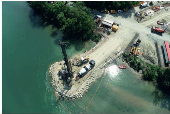
Fig. 6 Erstellung Pfeilerfundation mittels Furt. Construction of pier foundations using a ford.
