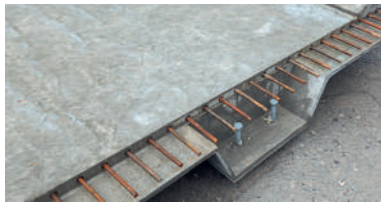
Fig. 7 Stossfuge zwischen zwei Trogelementen. Butt joint between two trough elements.
