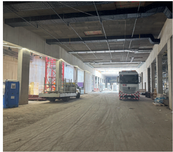
Fig. 7 Die 145 m lange Depothalle diente während des Baus dem Materialumschlag. The 145 m long depot hall was used for material handling during construction.
